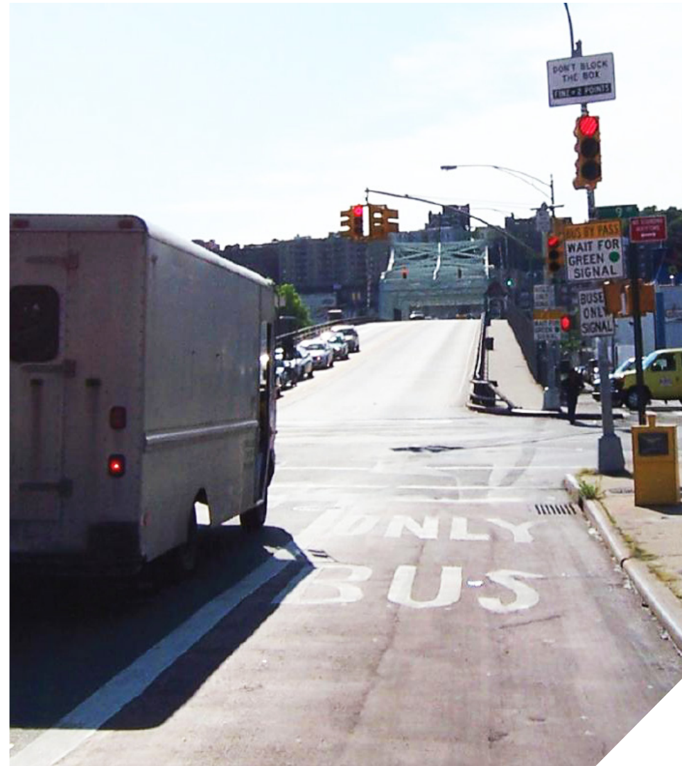
Figure 3-1 | Bus Only Lane / Leading Bus Interval, W 207th Street, Manhattan [Source: NYC Street Design Manual]
