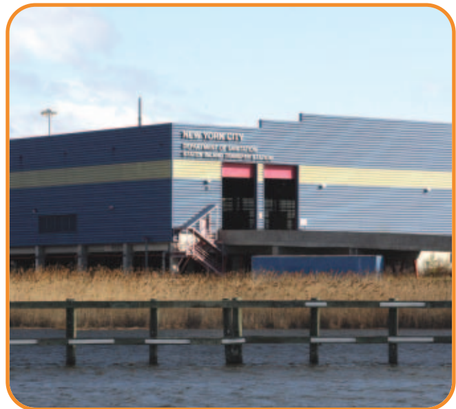
STATEN ISLAND TRANSFER STATION
