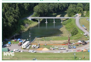
of Water Supply (BWS) are hitting the road again this week to discuss the ongoing, successful and nearly completed repairs downstream of Cannonsville Dam. Engineers have been working for weeks to repair boreholes that were drilled downstream of the dam to gather information for a hydroelectric facility planned for the site. The original boreholes tapped into a layer of pressurized groundwater and caused a cloudy discharge into the West Branch Delaware River in early July.
