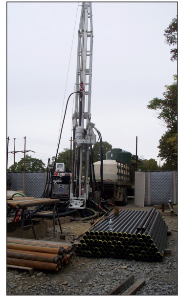
Coring Boring Machine
