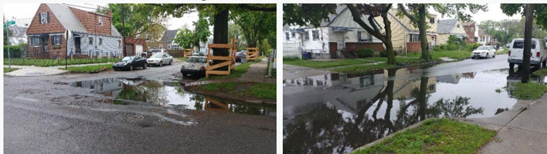
Examples of ponding in the project area following rain (May 2018)
