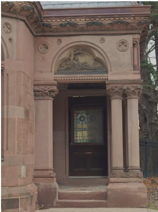
Porch to Ladies' Restroom, Visitors' Lounge Photo: Marianne Hurley, 2016
