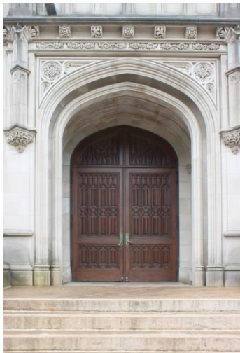
Entrance Portal, Chapel Photo: Sarah Moses, 2016
