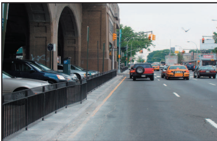
Pedestrian Fencing installed along parking facilities @ 47th Avenue and Queens Boulevard
