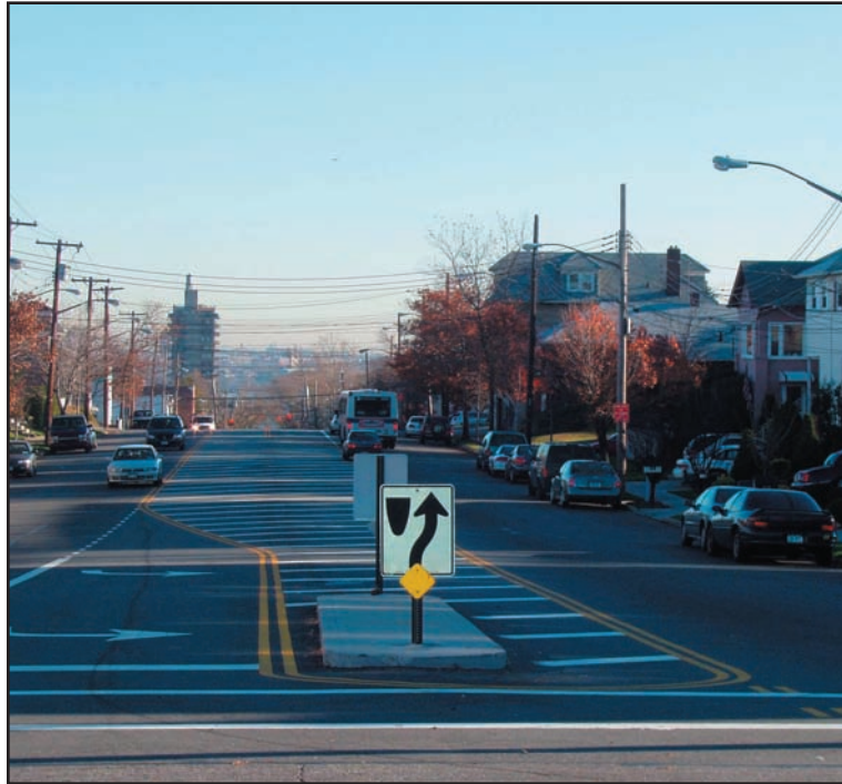
Roadway markings and raised intersection at Hylan Boulevard and Reynolds Avenue
