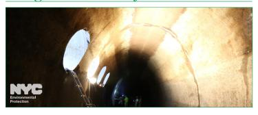
Construction continues at Delaware Aqueduct Shaft 4 in Ulster County, where DEP is working to connect the Delaware and Catskill aqueducts for the first time. Construction crews have already cored seven holes into the side of the Catskill Aqueduct, where they will install pipes in the coming months to make the connection. This will eventually allow DEP to move as much as 365 million gallons a day from the Delaware System into the Catskill Aqueduct.
