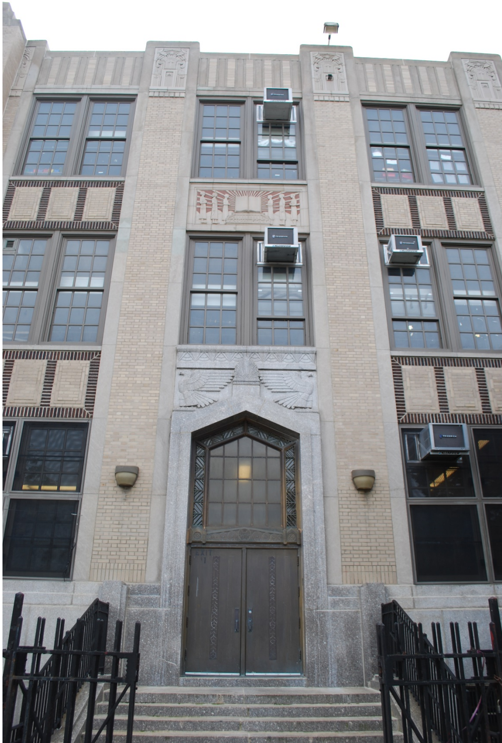
Public School 48, entrance with decorative details Michael Caratzas, September 2020
