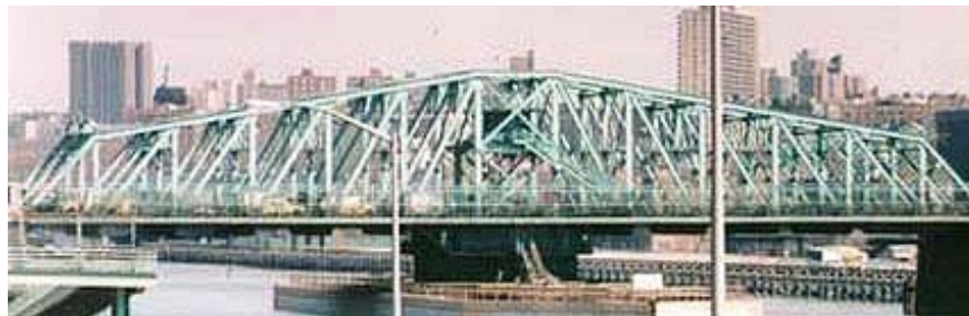
145 th Street Bridge
