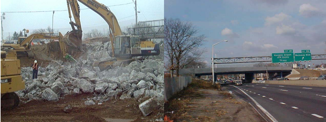
Demolishing the Old Guy Brewer Boulevard Bridge in March 2002
