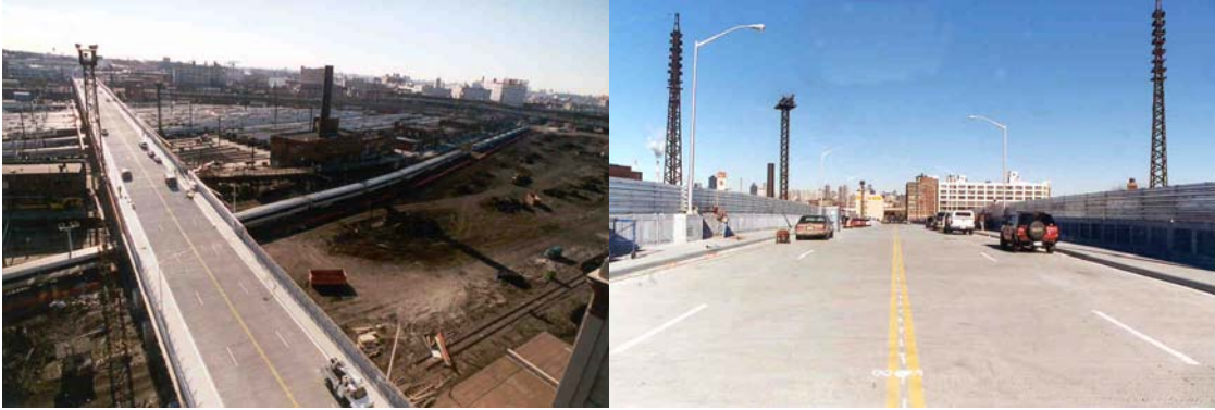
New Honeywell Street Bridge (Credit: Peter Basich)
