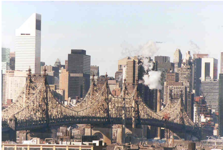
Queensboro Bridge (Credit: Peter Basich)
