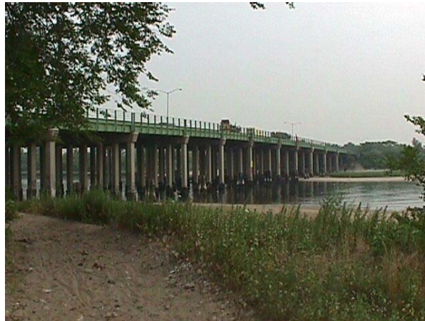
Paerdegat Basin Bridge
