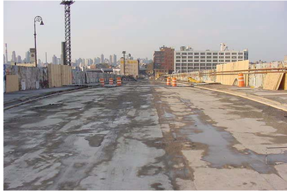
Old Honeywell Street Bridge Prior to Demolition
