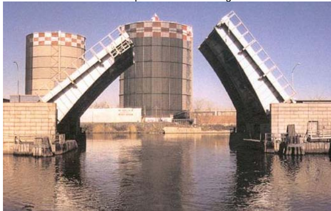
Metropolitan Avenue Bridge
