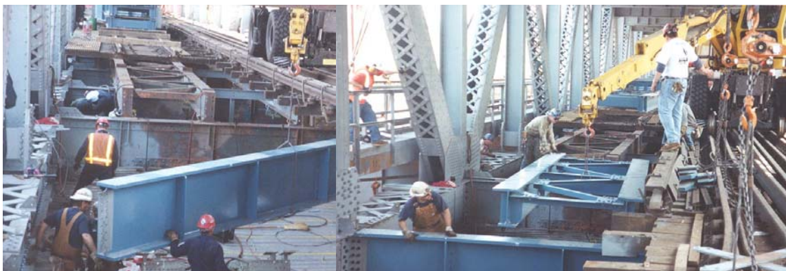
Installation of New Floorbeams & Stringer Panels for the Subway Support Steel
