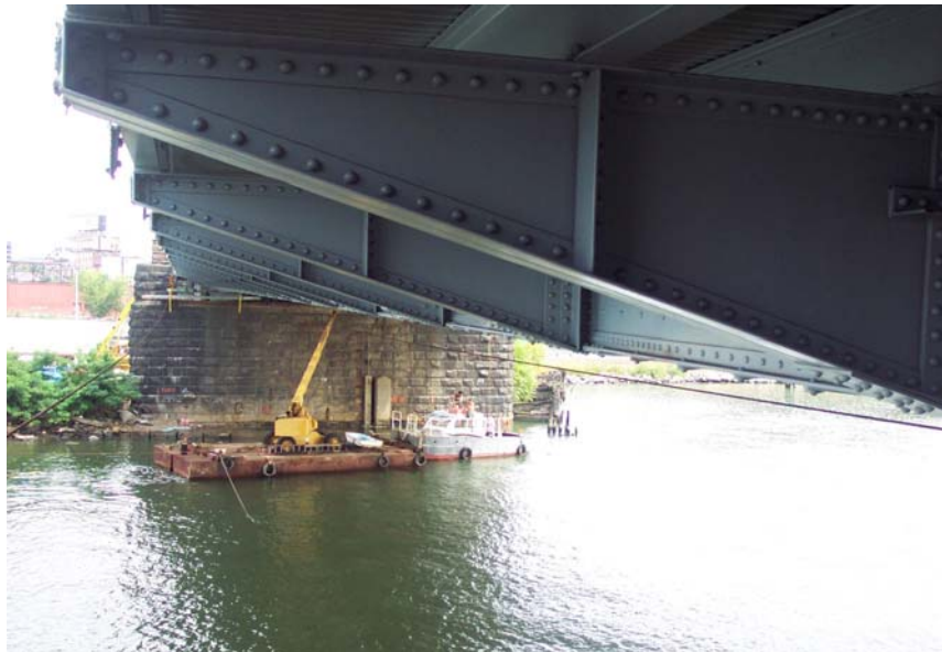
Bridge Inspectors in Bucket Truck under the Willis Avenue Bridge (Credit: Bojidar Yanev)
