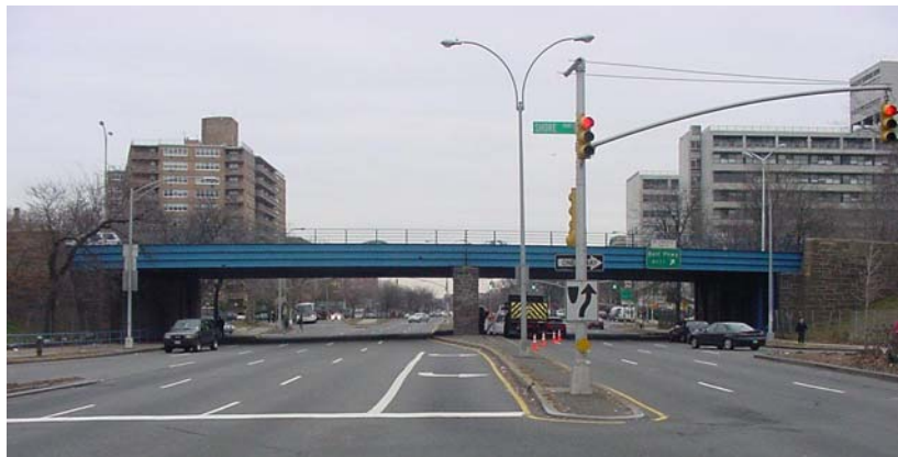
Current Belt Parkway Bridge Over Ocean Parkway
