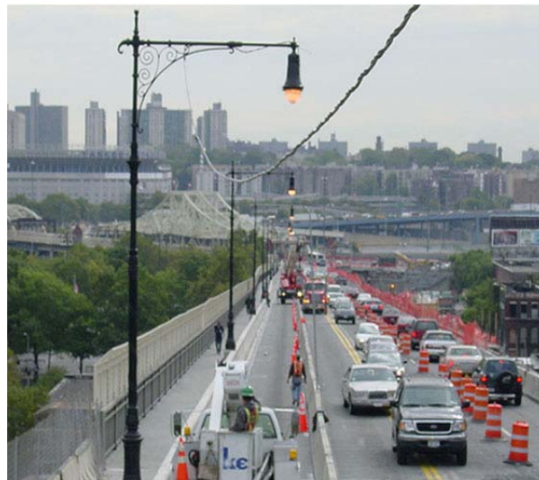
West 155th Street Viaduct of the Macombs Dam Bridge
