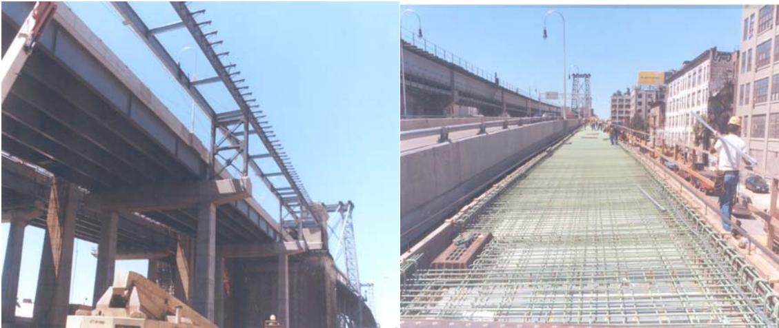
Contract #7 Bikeway Steel Erection & Rebar Installation
