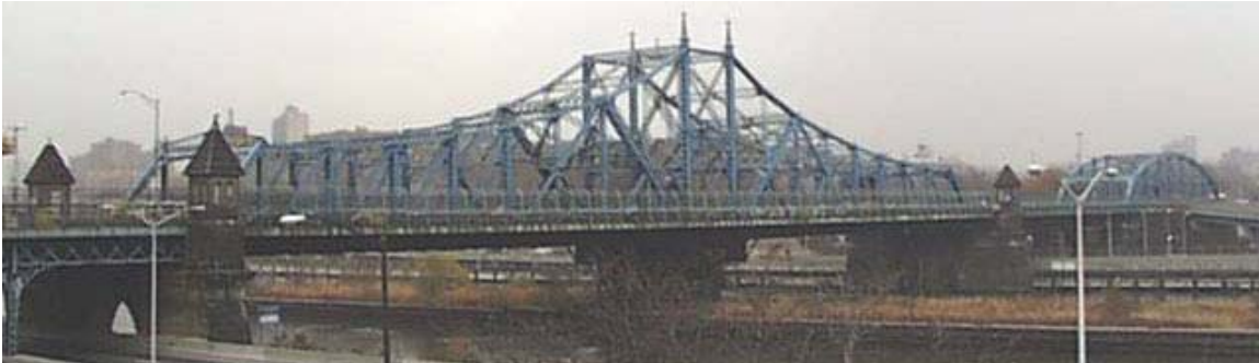
Macombs Dam Bridge
