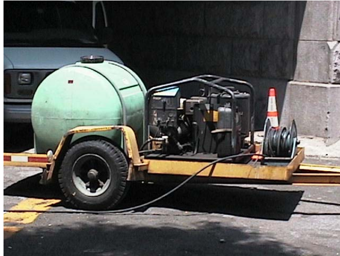
Pressure Washing Machine Used for Graffiti Removal. It is Set to 2500 psi and 212° F.
