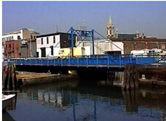
Carroll Street Bridge Over the Gowanus Canal
