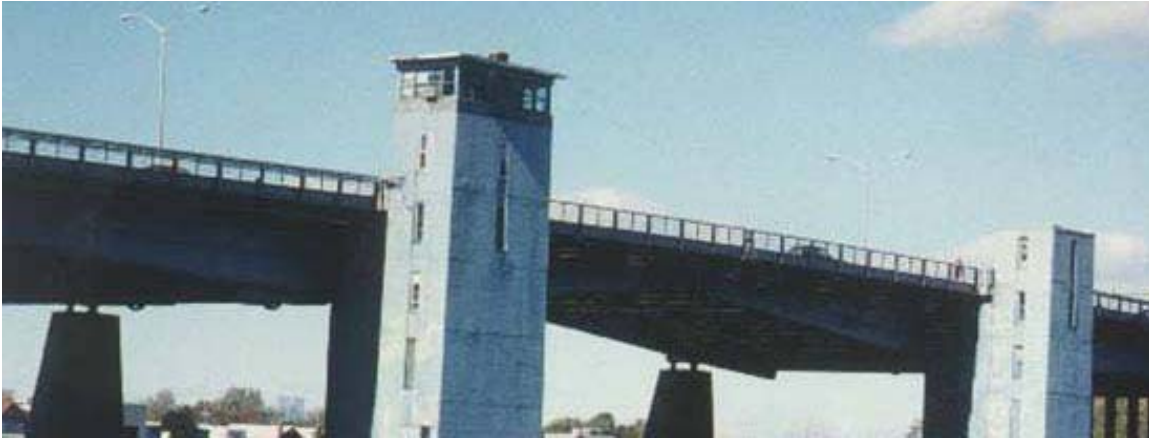
Mill Basin Bridge
