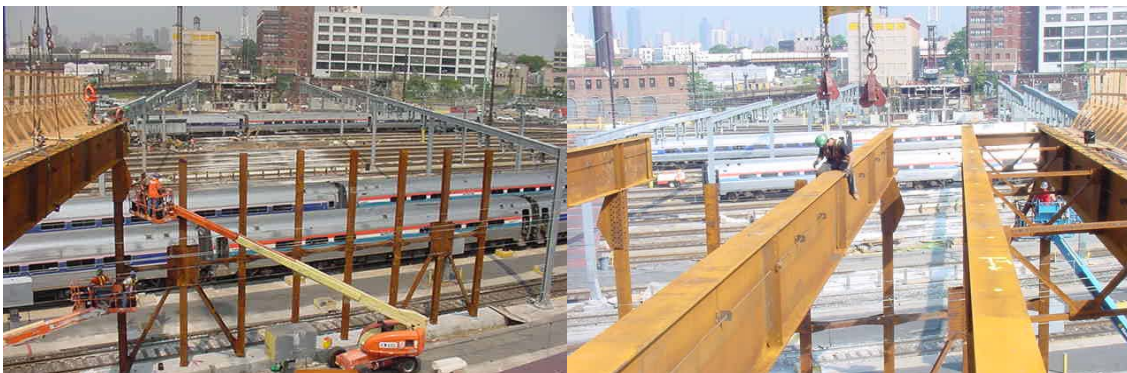
Structural Steel Erection of Span #9 of the New Honeywell Street Bridge
