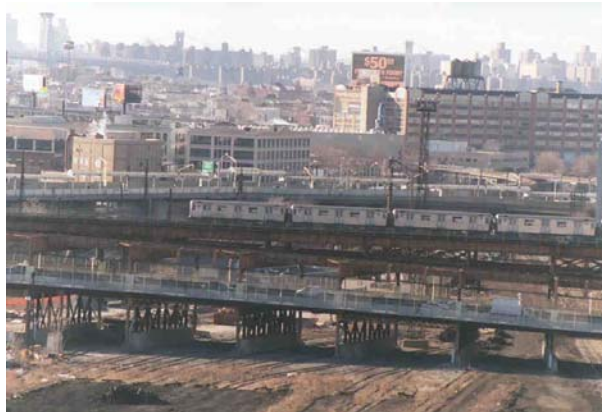
Reconstructed Queens Boulevard Bridge (Credit: Peter Basich)
