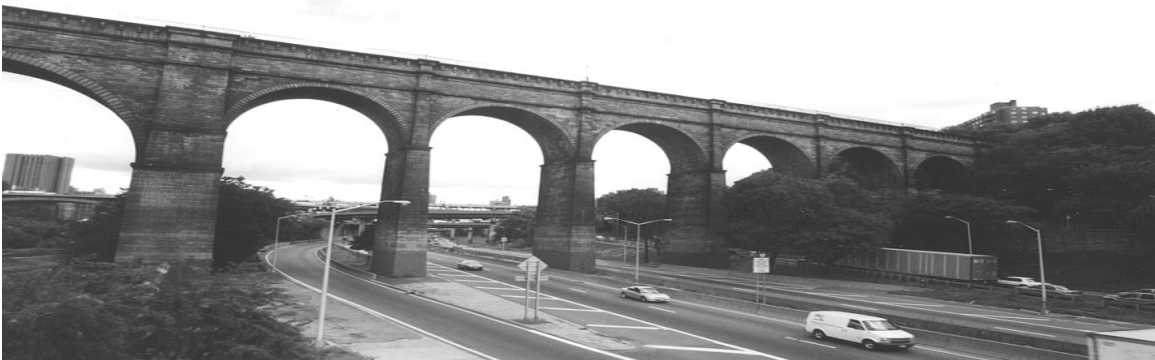
High Bridge Pedestrian Bridge (Credit: Peter Basich)
