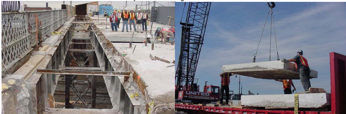
Removal of Old Honeywell Street Bridge Deck Slabs
