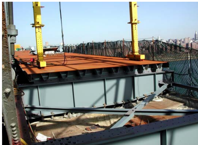
Contract #7 Installing An Orthotropic Deck Panel
