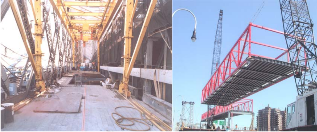
Contract #7 Replacing the North Inner Roadway Deck & Erecting the Footwalk
