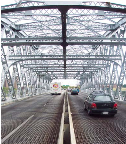
Willis Avenue Bridge Grating (Credit: Bojidar Yanev)
