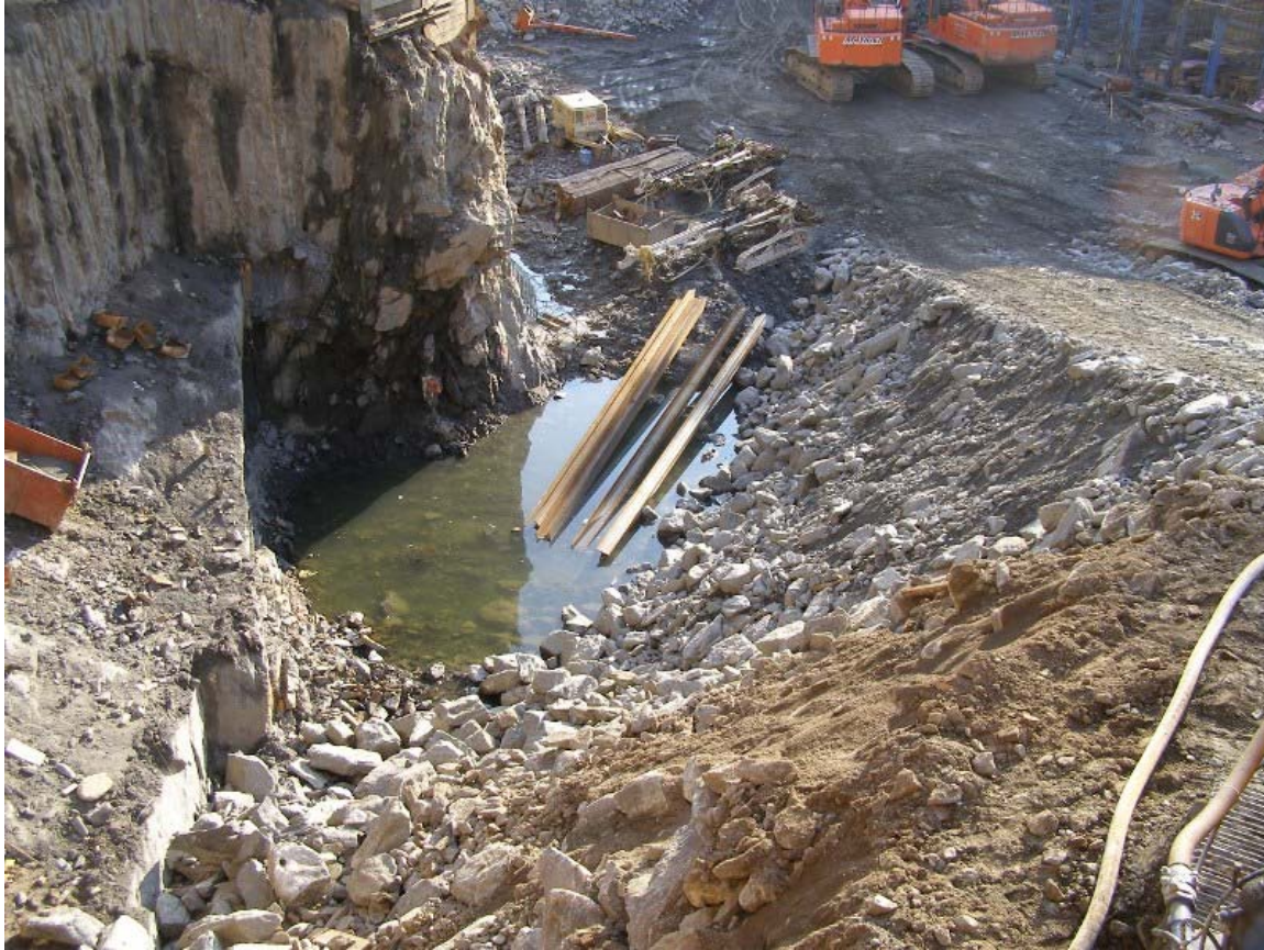
Photo 10 – Face of Rock after Blasting on 7/25/07
