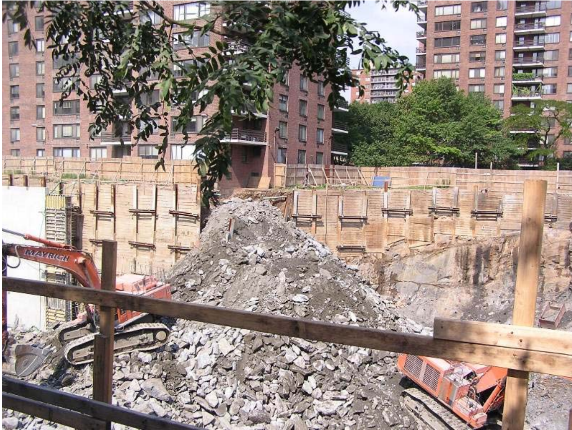
Photo 3 – Stabilization –Earthen Berm
