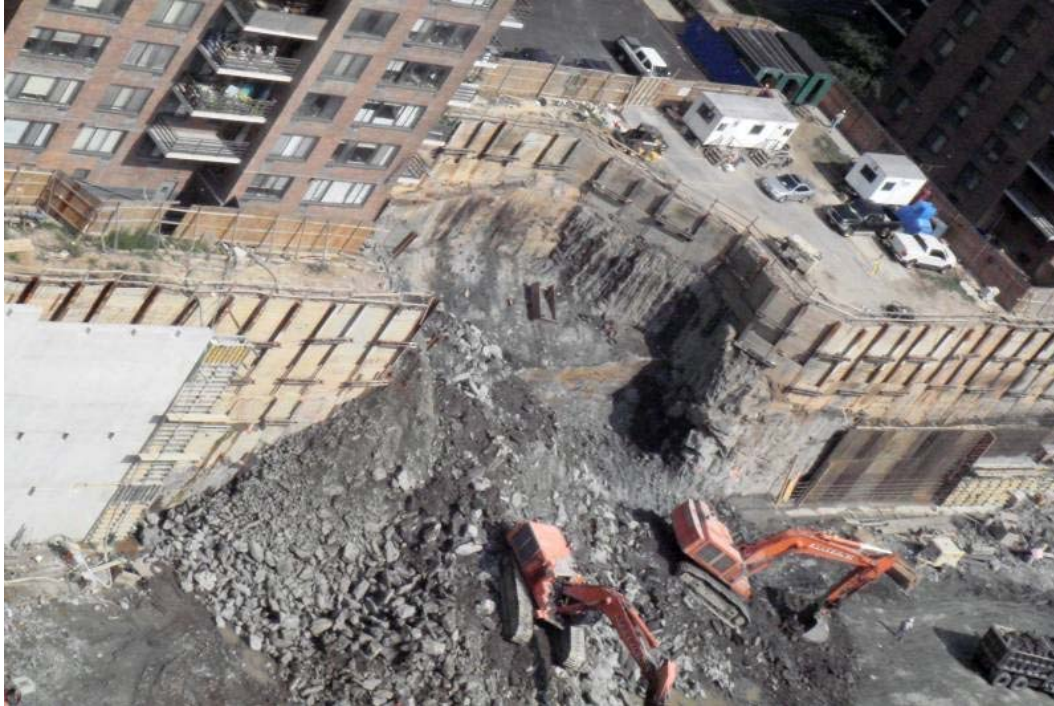
Photo 2 – Stabilization Berm
