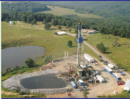
This picture shows a typical Drill/Well Pad with associated drilling rigs, storage, treatment, roads and waste management facilities. Source: Rapid Impact Assessment Report September 2009
