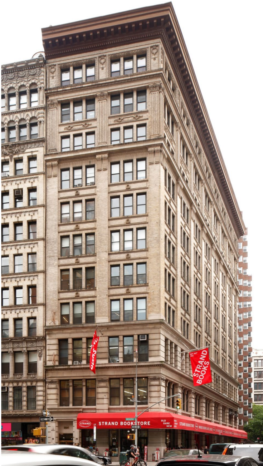
826 Broadway Building (now the Strand Building) Sarah Moses, June 2019
