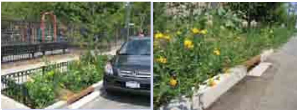
An enhanced tree pit, left, and swale, right, manage stormwater efficiently and also green neighborhoods.
