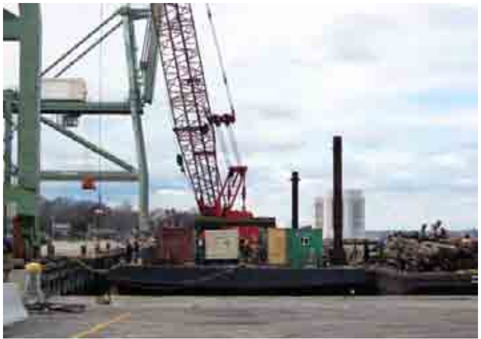
Repairing fendering and piles at Pier 9A North at the Red Hook Container Terminal.
