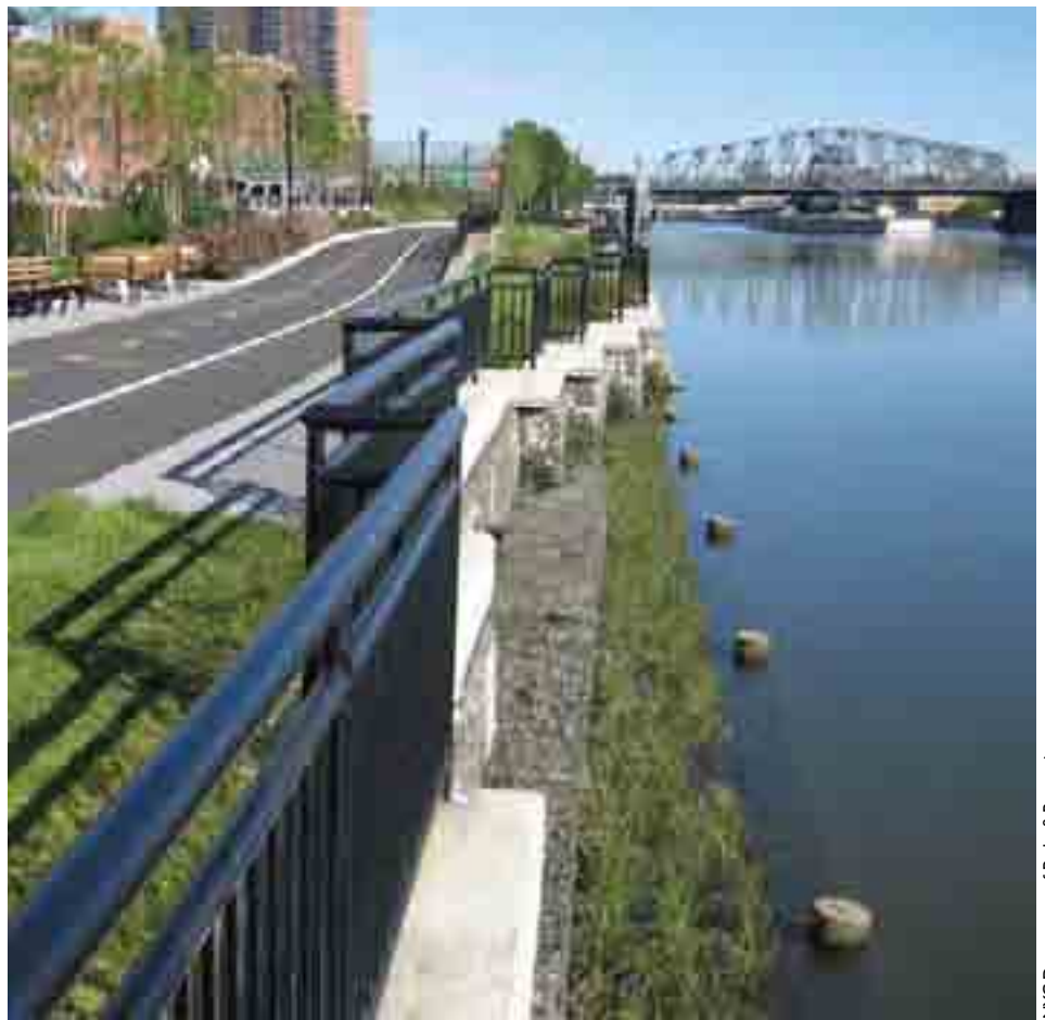
The seawall at Harlem River Park features stepped gabions planted with salt marsh grasses.
