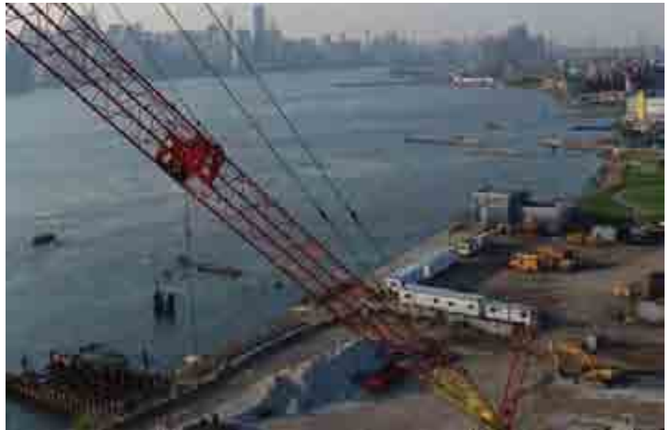
Redevelopment under way on the Williamsburg waterfront.
