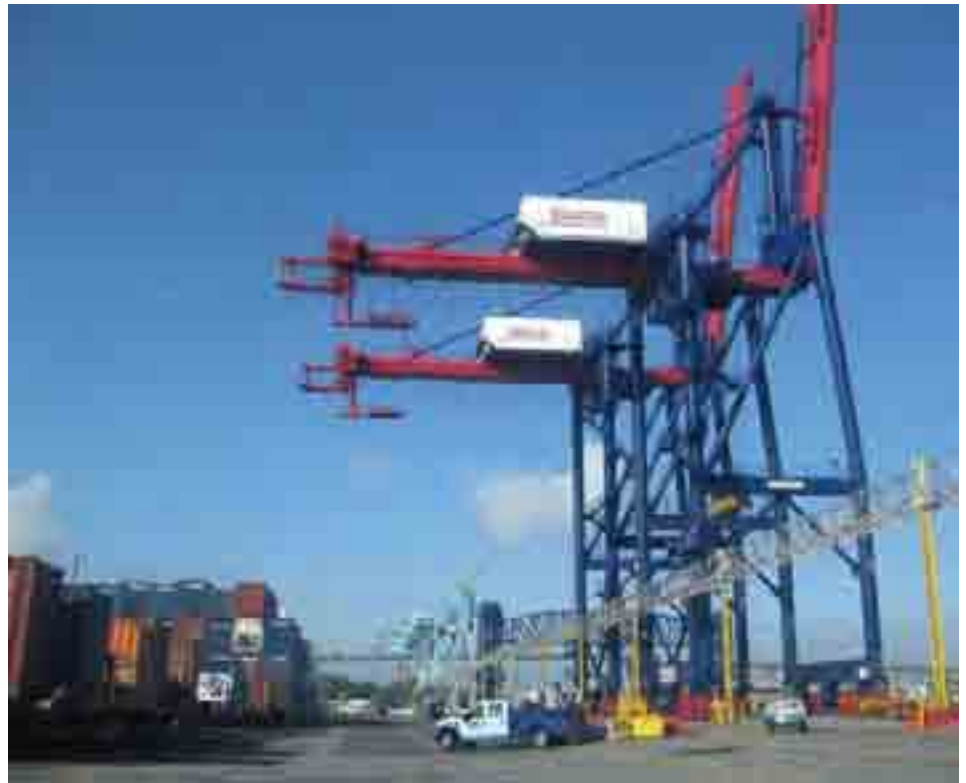
New York Container Terminal on Staten Island.
