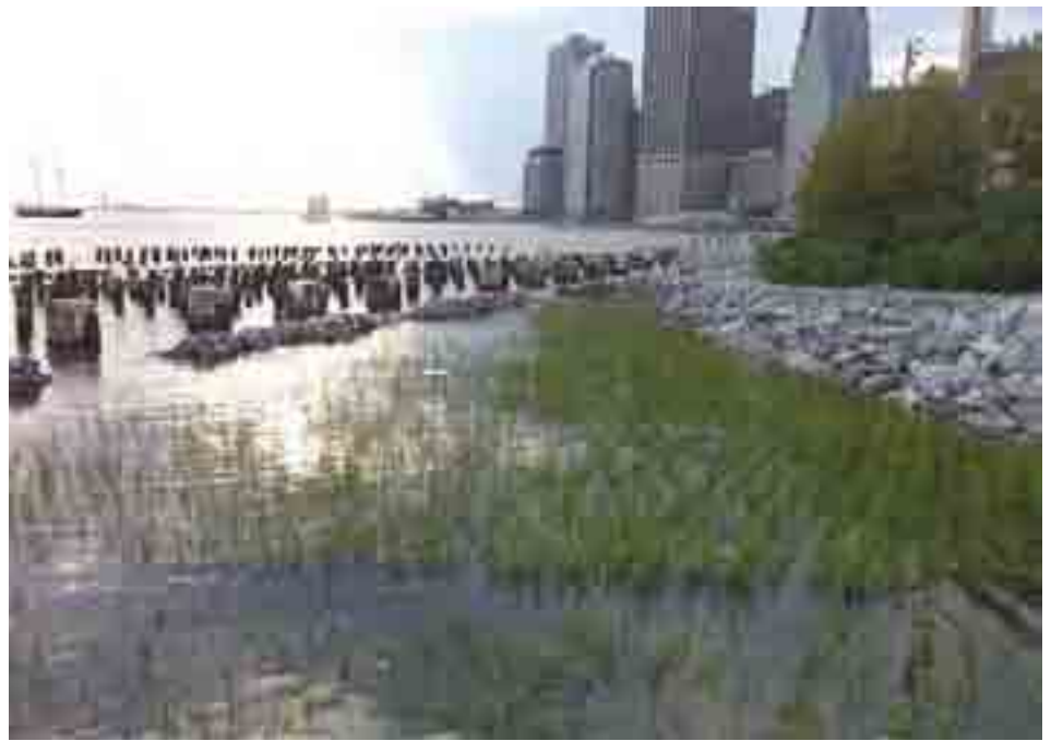
“Soft edges” deployed at Brooklyn Bridge Park are part of the site’s stormwater management system. The constructed wetland also dissipates wakes and provides habitat.
