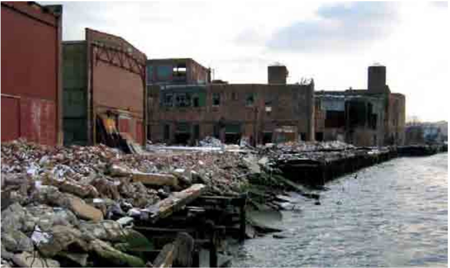
The Greenpoint Terminal Market site on the Brooklyn waterfront.
