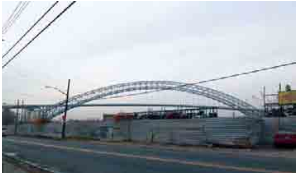
Opaque fences block views on Staten Island's North Shore.
