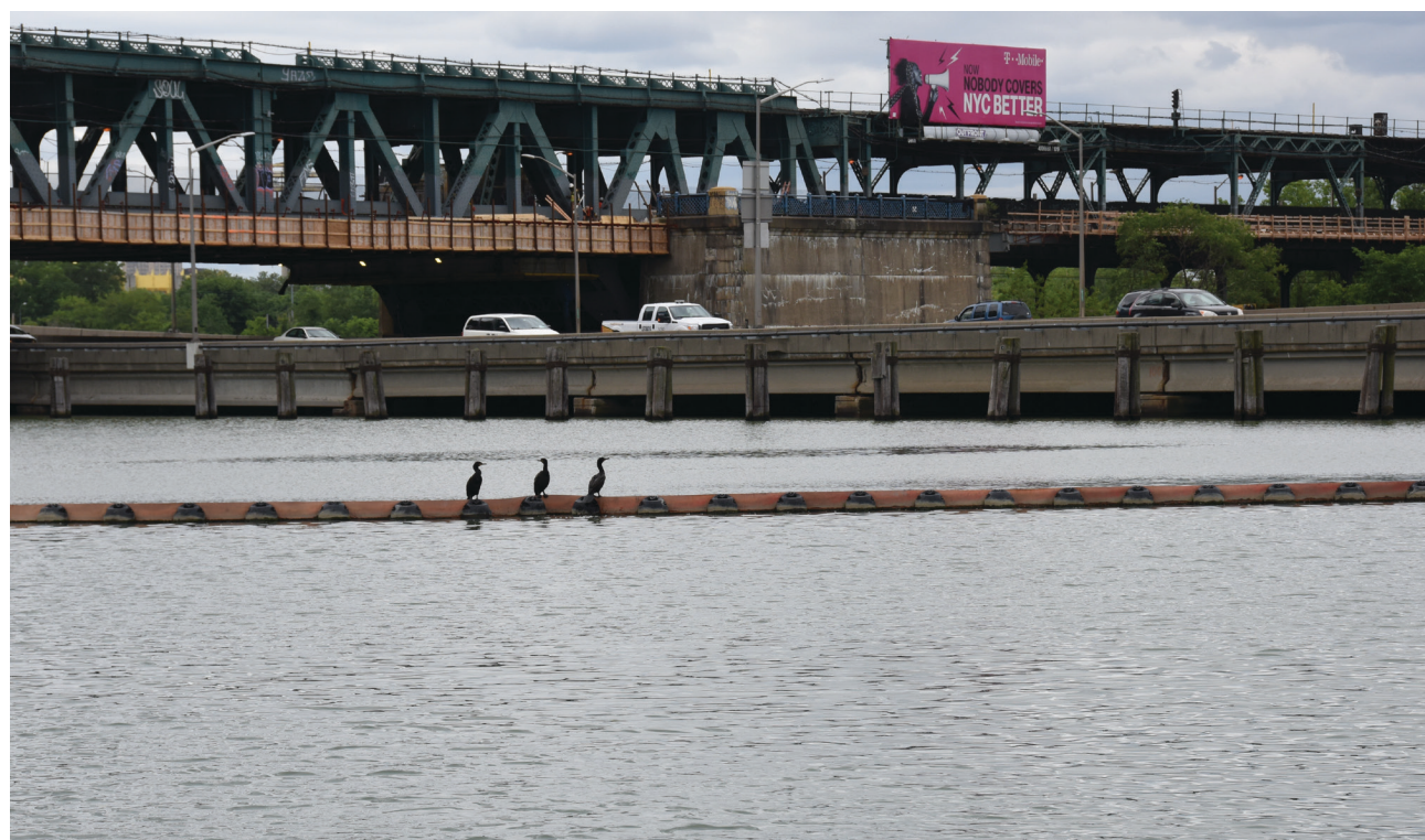
Floating Boom in Flushing Creek
