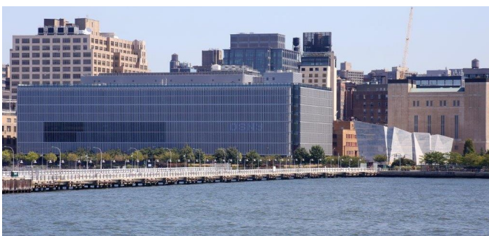
The Manhattan 1/2/5 garage and Spring Street salt shed.
