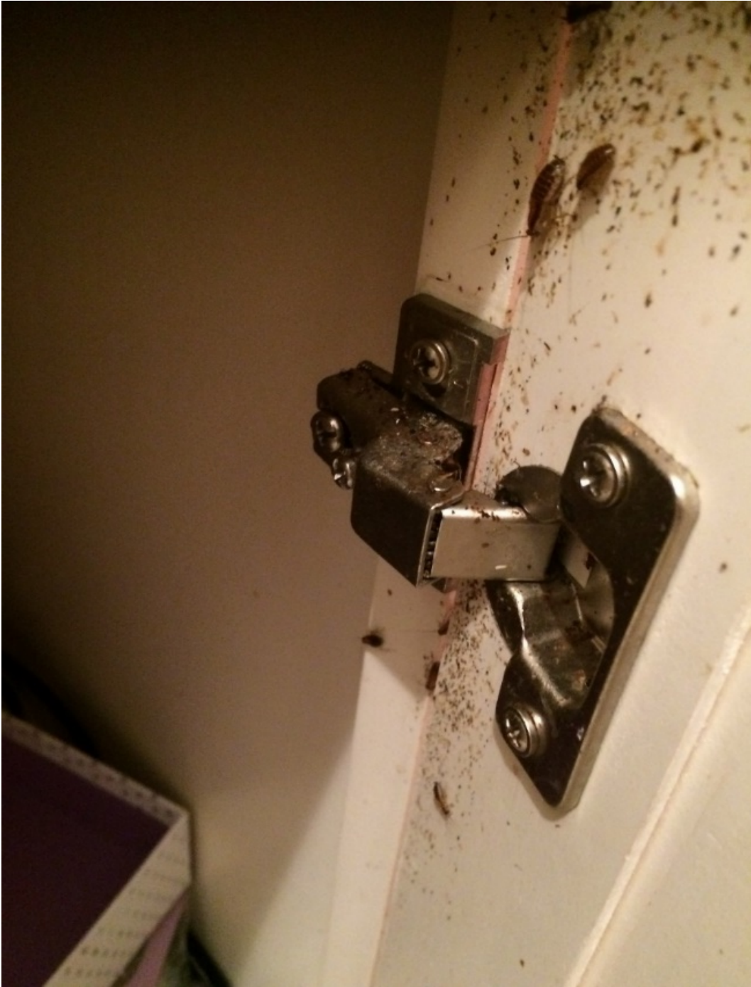
Photo 9 - Roaches Crawling Out of Kitchen Cabinet
