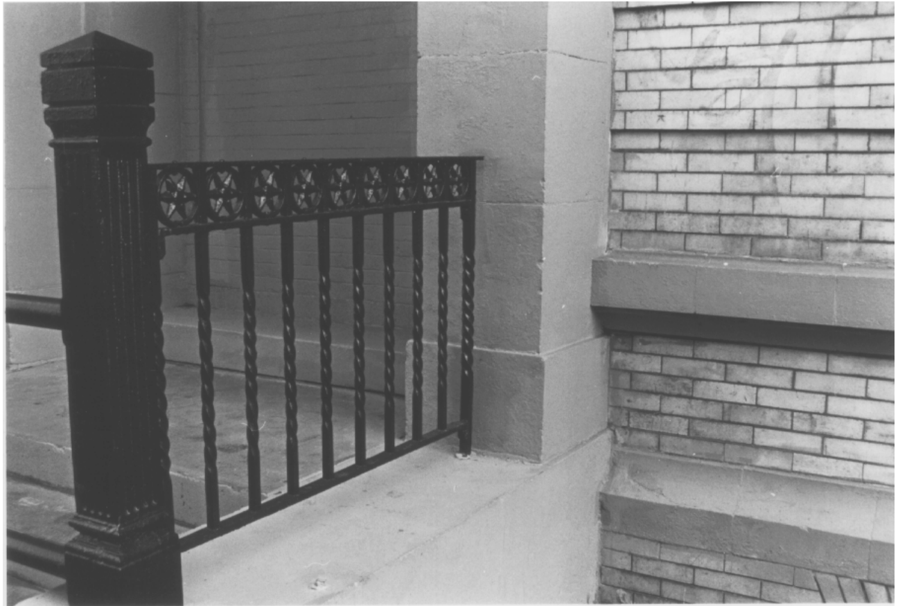
Fig. 15 Bowling Green Offices, Detail of ironwork on Greenwich Street
