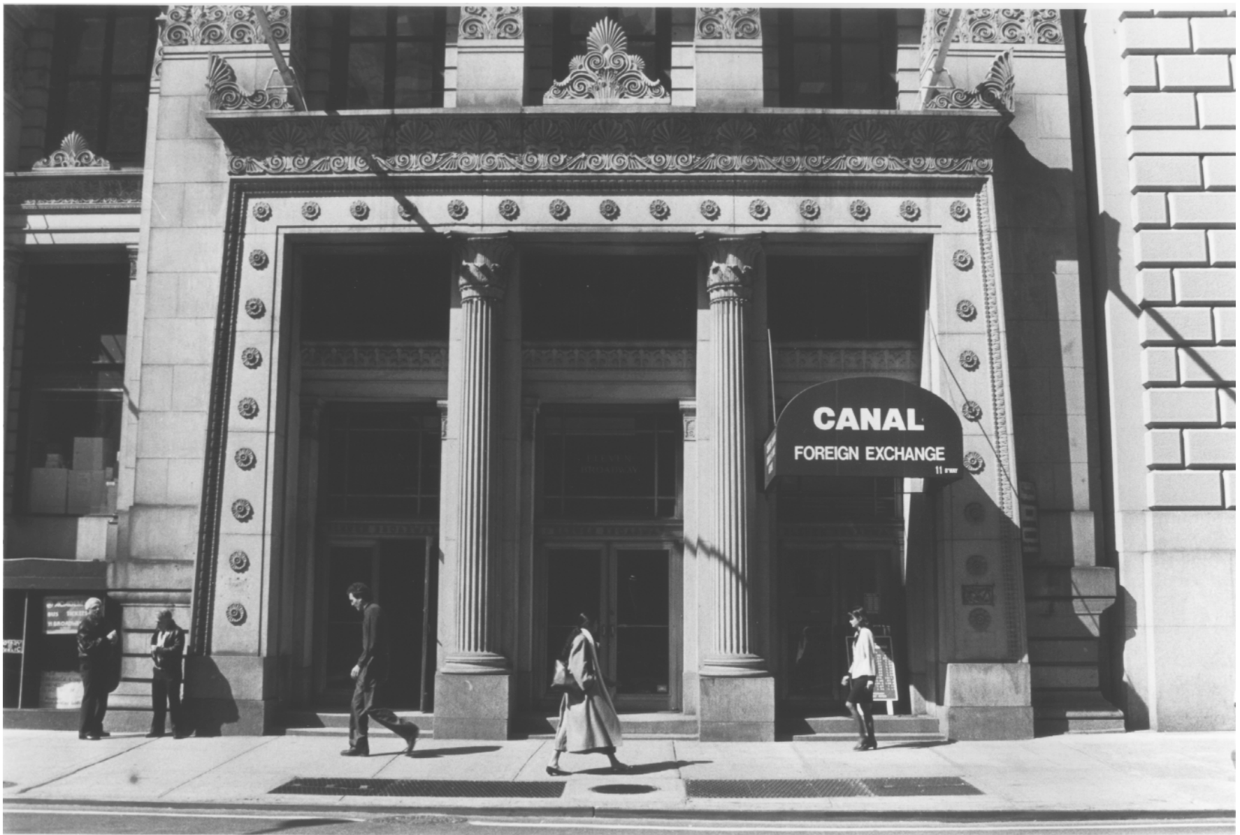
Fig. 6 Bowling Green Offices Building, 5-11 Broadway, North portico on Broadway
