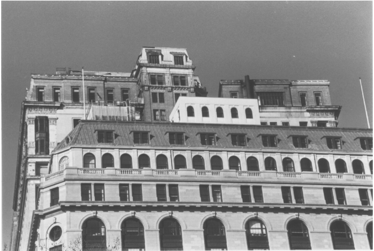
Fig. 16 Bowling Green Offices, South elevation (part of No. 1 Broadway in foreground)
