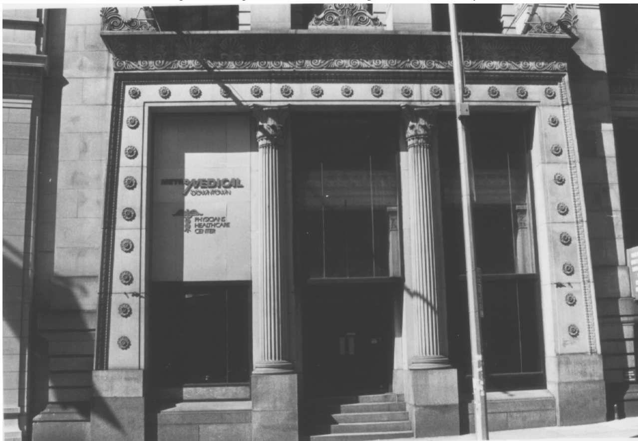
Fig. 8 Bowling Green Offices, South portico on Broadway
