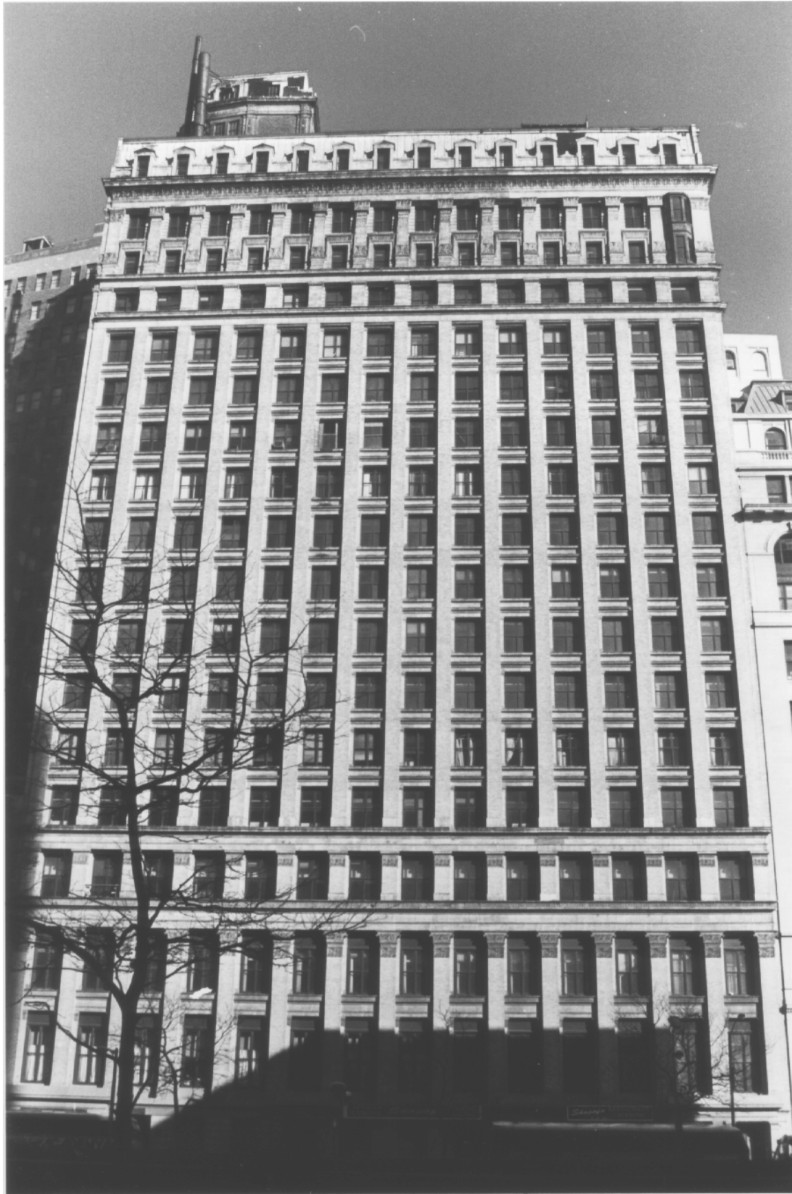
Fig. 11 Bowling Green Offices Building, 5-11 Broadway, Greenwich Street facade
