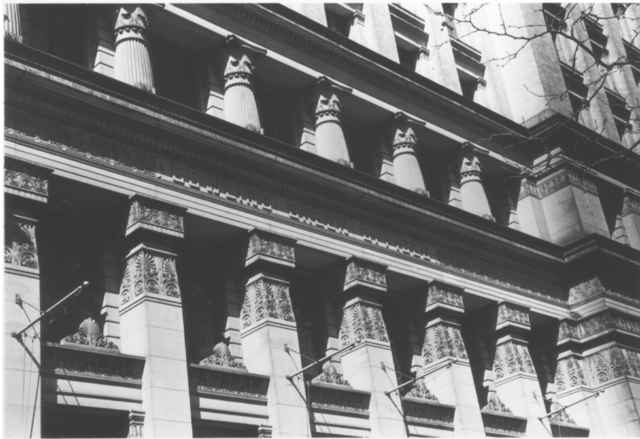
Fig. 7 Bowling Green Offices, Detail of second-third stories facing Broadway Photos: DMB
