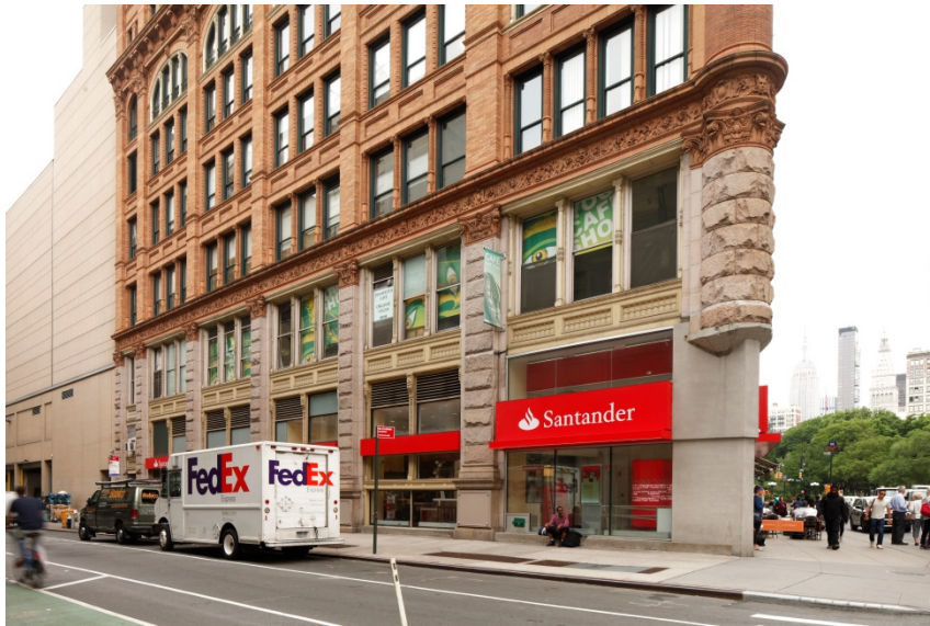
13th Street Facade, The Roosevelt Building Sarah Moses, June, 2019
