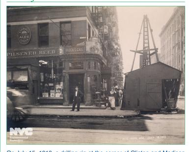
On July 15, 1910, a drilling rig at the corner of Clinton and Madison Streets on the Lower East Side makes borings to discover geological conditions far below the pavement in preparation for City Water Tunnel No. 1. Photographs like this give a glimpse into the past and provide a peek at buildings lost to time and development—Gouverneur Hospital was built on this block in 1972.
