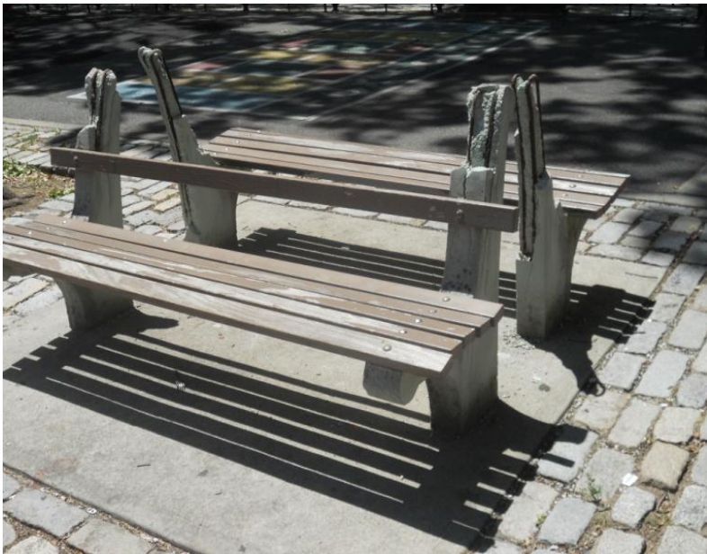
14. Fox Playground Broken benches
