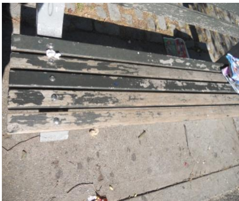
2. Brighton Playground Peeling paint on benches
