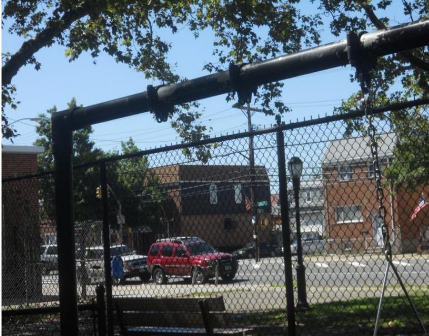
3. Dr. John's Playground Missing swings
