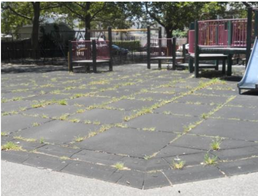
8. Jacob Joffe Playground Heavy weeds at playground
