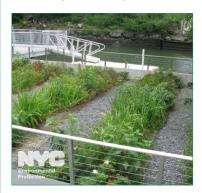
Construction of this prototype green infrastructure park included excavating the roadway to a depth of five feet and installing a modular system of concrete cells filled with engineered soil to store and filter stormwater runoff. Native, mostly woody, plants absorb, filter and evapotranspirate water through their roots and leaves, as well as act to phyto-remediate toxins from the runoff. A ten
