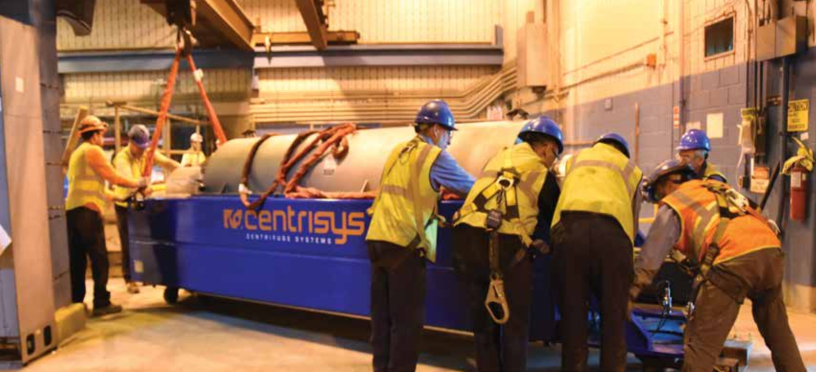
Centrifuge Installation at Hunts Point Wastewater Treatment Plant
