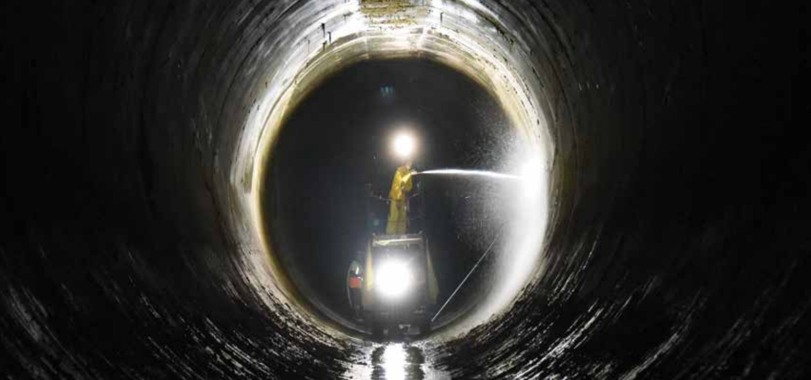
City Water Tunnel No. 3
