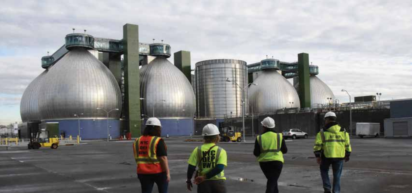
Newtown Creek Wastewater Treatment Plant
