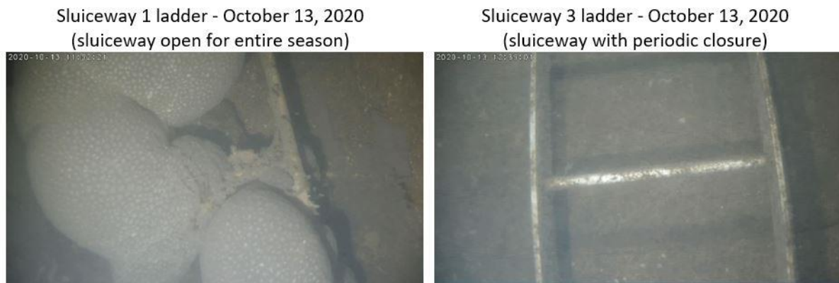
Figure 4.8 Comparison photos of Shaft 18 sluiceways 1 and 3 showing the size and condition of P. magnifica on October 13, 2020. For scale, each of the ladder rungs is about 12 inches across.
