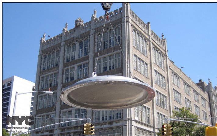
New Shaft Cap being delivered for Shaft Rehabilitation Project, Manhattan, NY (9/13/12)
