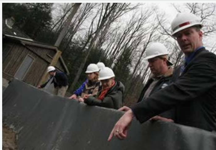
DEP engineer Sean McAndrew (right, pointing) shows Commissioner Emily Lloyd (center) some of the work that was done to wake the Ashokan Release Channel ready for use. In this area barricades were erected to direct the flow of water away from buildings that are part of the Ashokan Field Campus. Up to 600 million gallons of water per day will flow through the channel from the Ashokan Reservoir in order to decrease the chance of flooding in downstream communities along the lower Esopus Creek.
