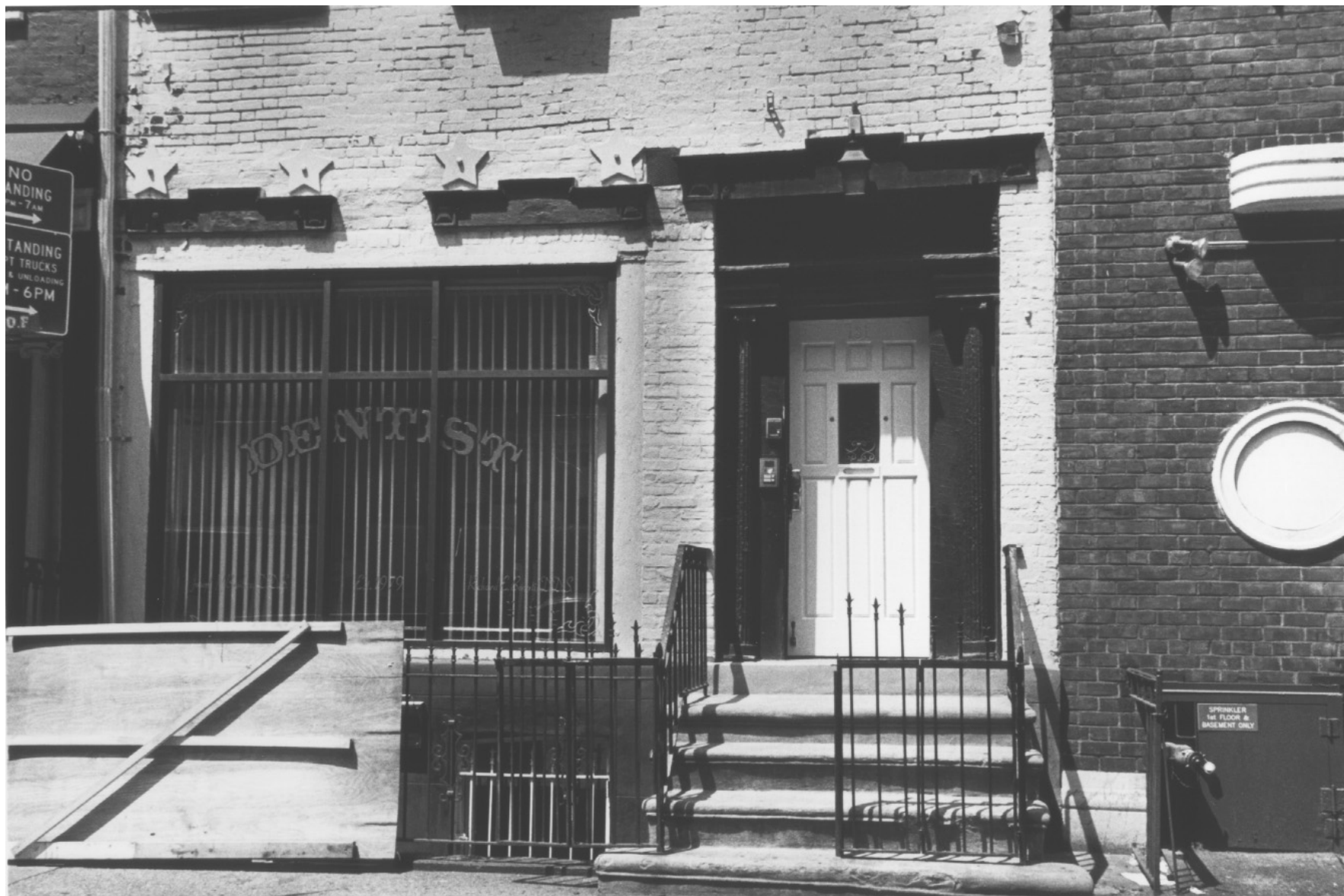
131 MacDougal Street House, first story Photo: Carl Forster
