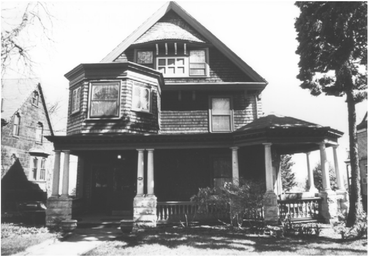
231 St. Paul's Avenue Built: 1888. Architect: Not Determined
