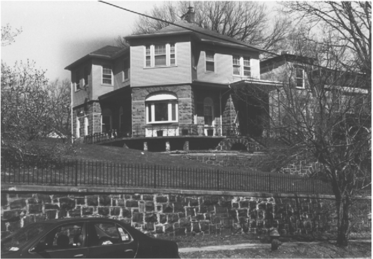
368 St. Paul's Avenue Built: c. 1891 with later alterations. Architect: attributed to Paul Kuhne.
