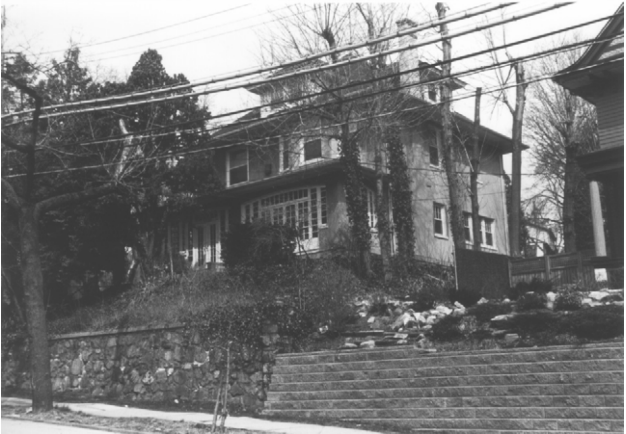
147 Cebra Avenue Built: 1915-17. Architect: attributed to Henry G. Otto.
