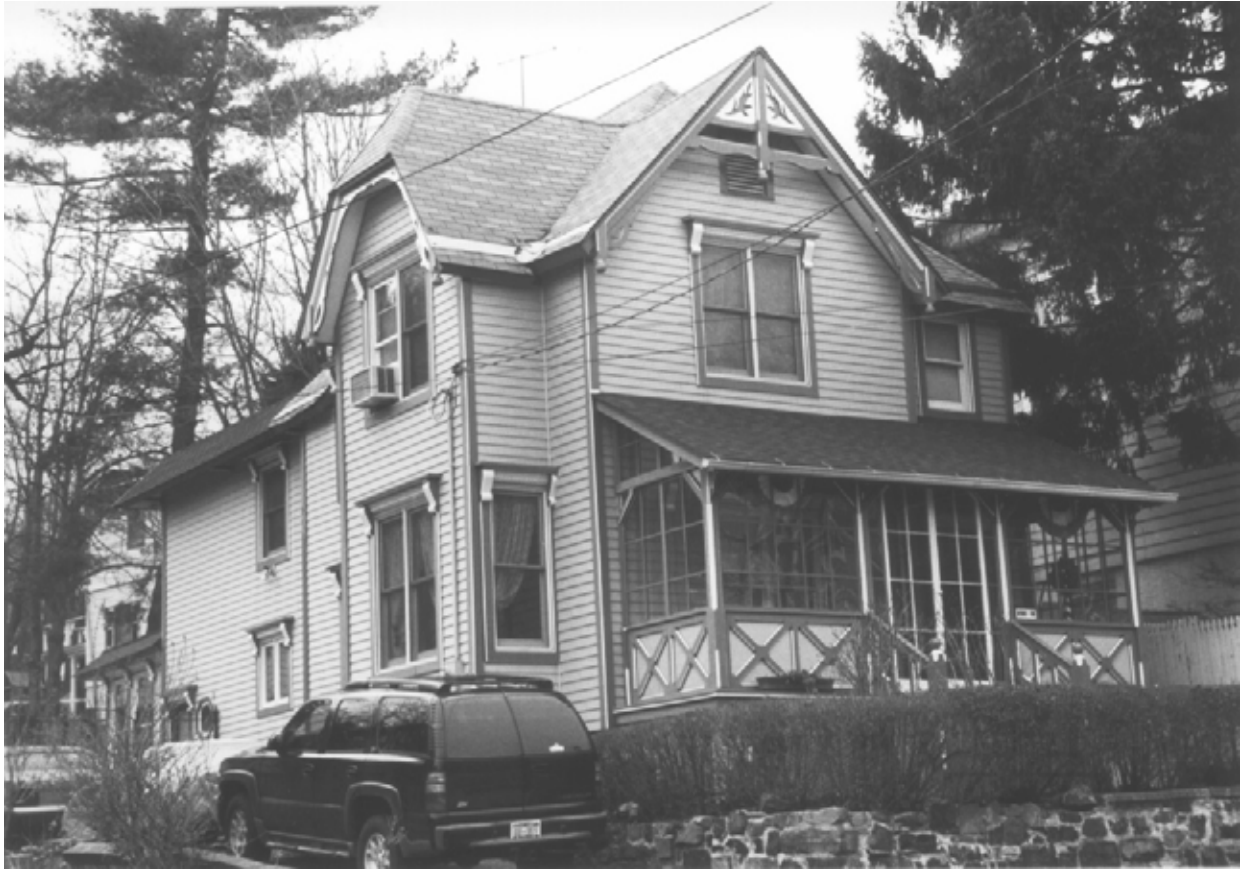
194 Cebra Avenue Built: c. 1881-82. Architect: Not Determined
