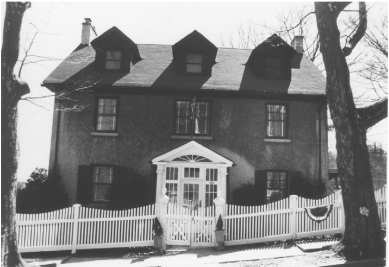
131 Marion Avenue Built: 1992. Architect: Otto Loeffler.
