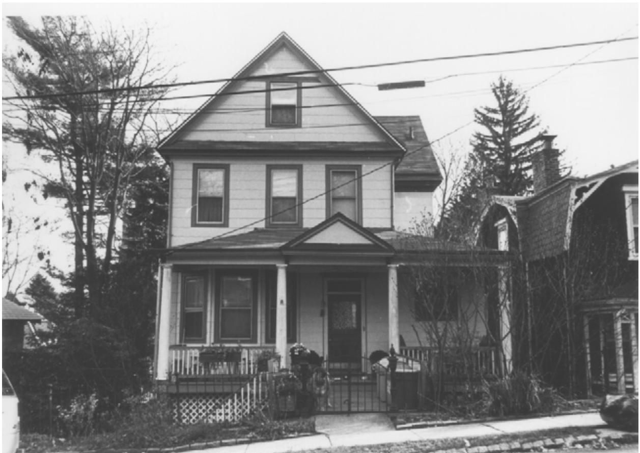
17 Marion Avenue Built: 1907. Architect: Conrad L. Larsen.
