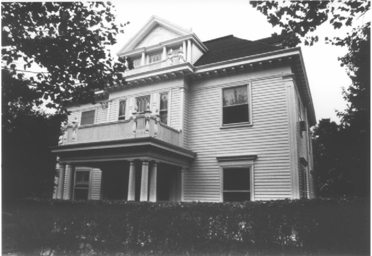
91 Marion Avenue Built: 1899-1900. Architect: Otto Loeffler.
