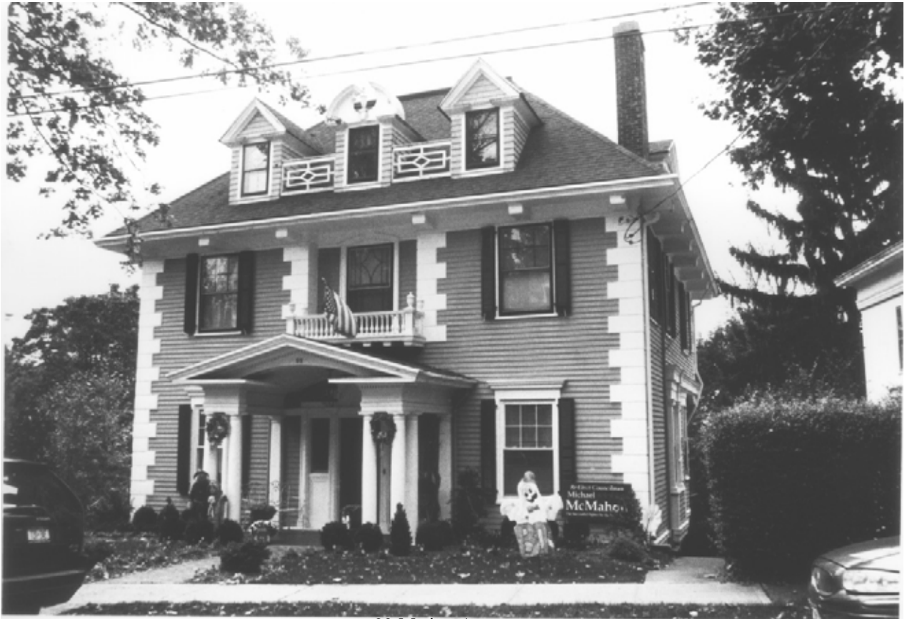
99 Marion Avenue Built: 1907-08. Architect: Otto Loeffler.
