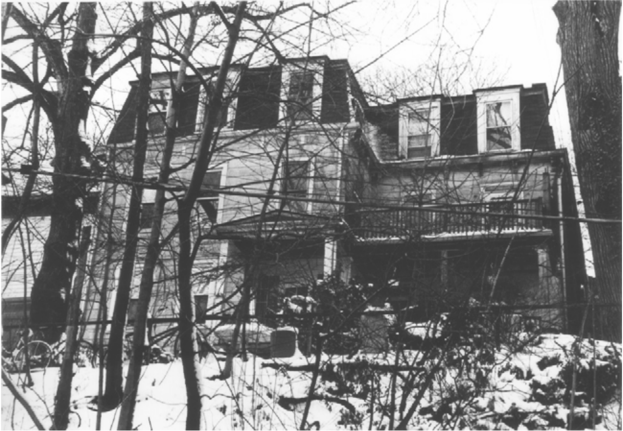
210-212 St. Paul's Avenue Built: 1855-60. Architect: Not Determined
