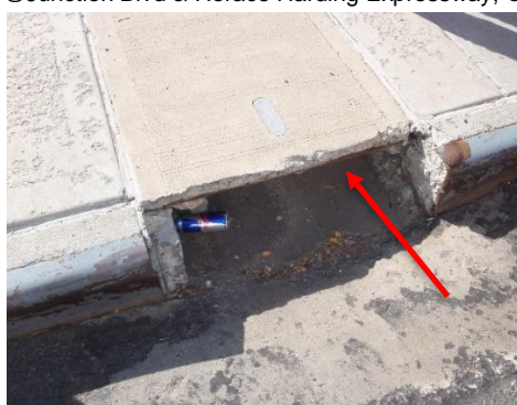
Broken concrete edging with exposed rebar* @Junction Blvd & Horace Harding Expressway, Queens
