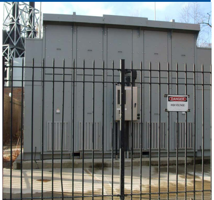
Fencing surrounding the outdoor Electrical Substation
