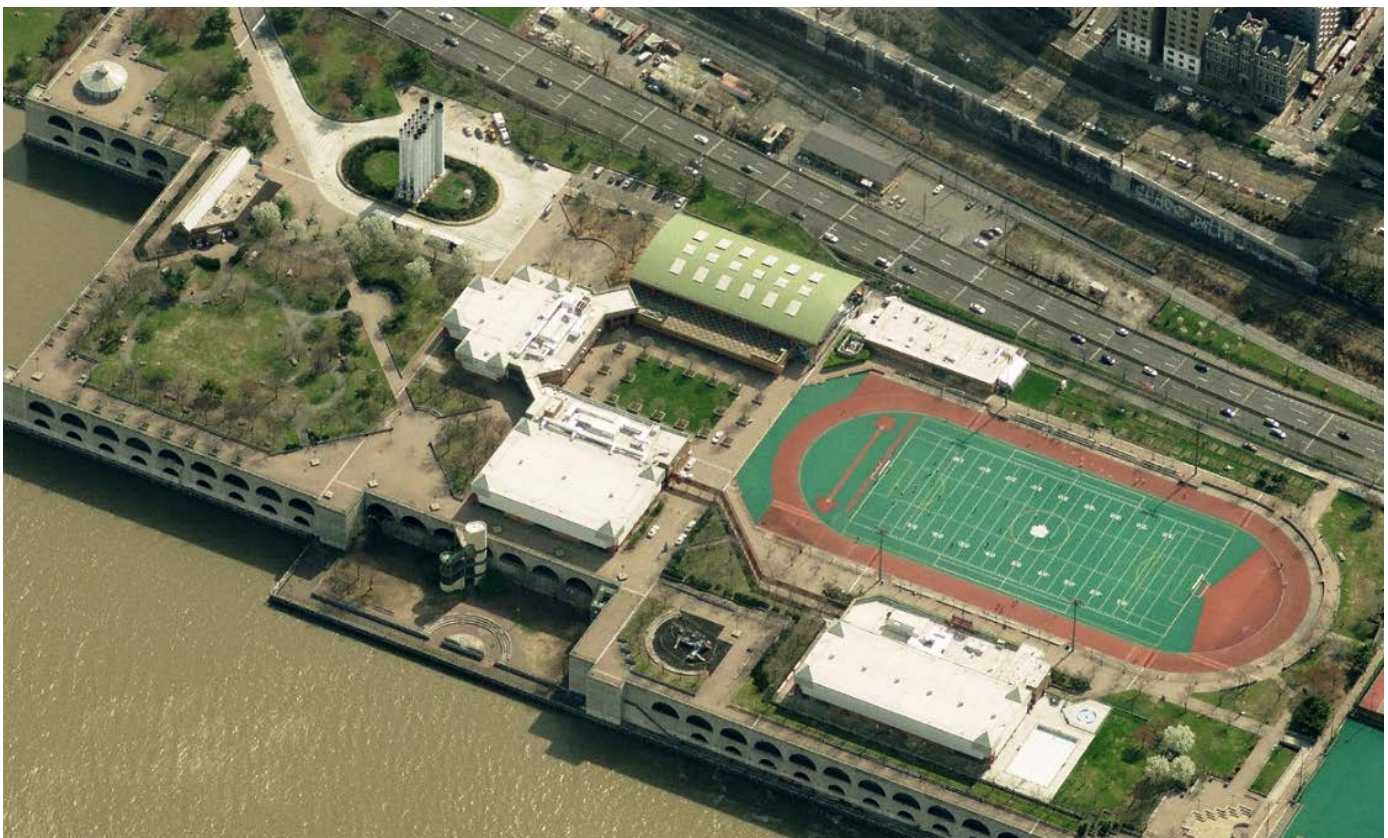
North River Wastewater Treatment Plant
