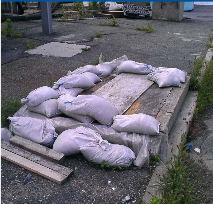
The overhead grate above the Aeration Gallery is a potential flood pathway to the sludge pumps.
