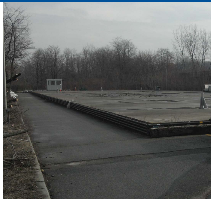
Chlorine Contact Tanks are potentially at risk of flooding during a large storm event.
