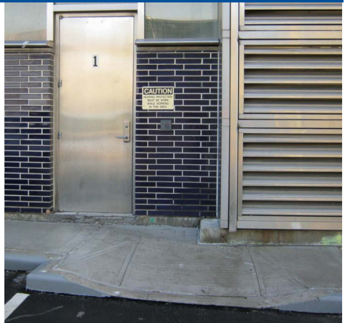
Low-lying louvers along-side the Main Building
