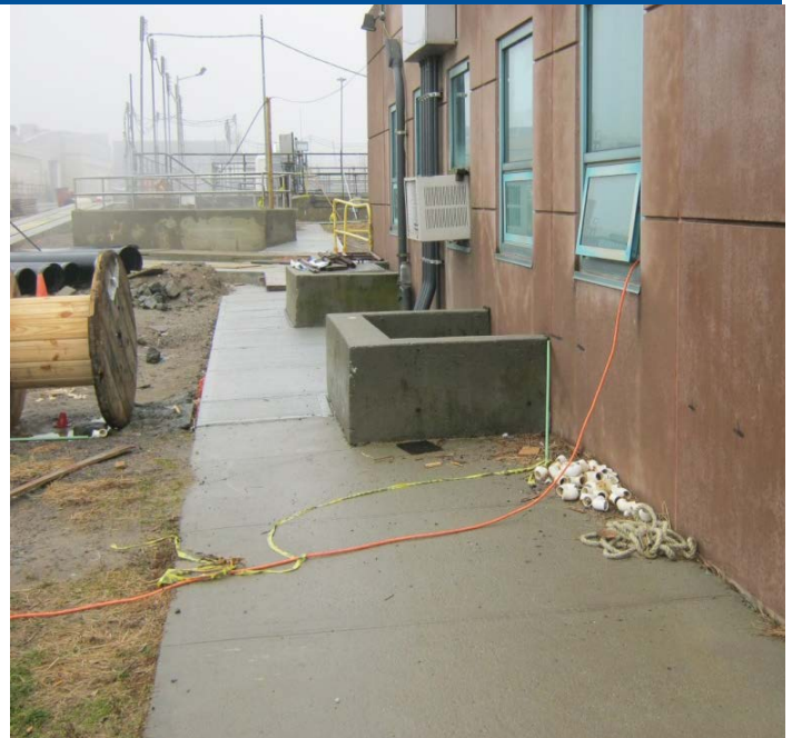
Basement access ways into the Chlorine Building
