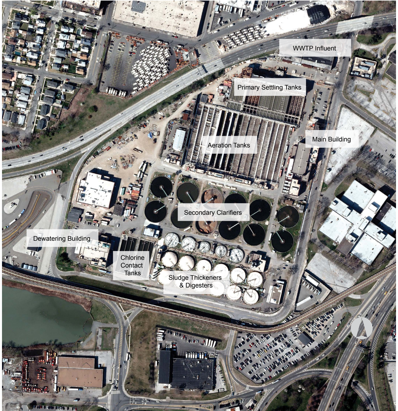
The Jamaica Wastewater Treatment Plant did not sustain any damage due to flooding during Hurricane Sandy.
