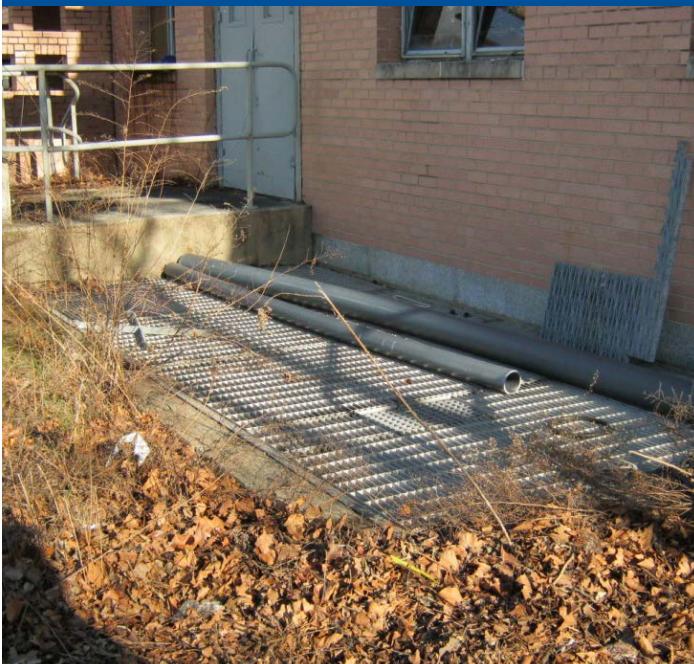
Floor grate outside of the Maintenance Building
