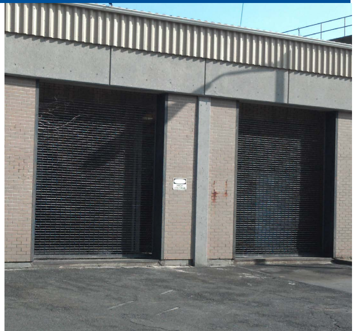
Rollup doors at the Electrical Substation Building
