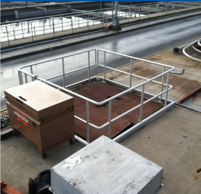
Typical hatch at grade level leading to tunnel system
