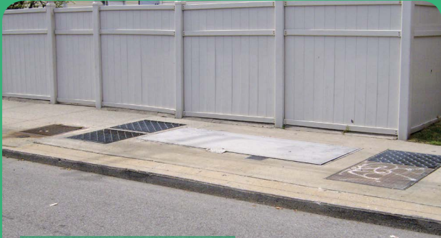
Avenue M: Under the sidewalk
