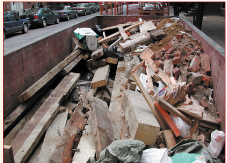
DOS collects around 600,000 tons of construction and demolition debris from City building projects each year. None of this is counted towards the City’s recycling rate.
