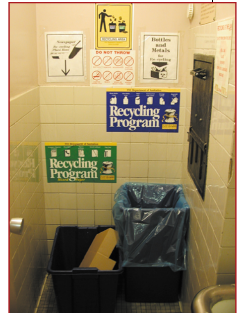
This garbage chute is typical of larger apartment buildings constructed in the mid to late 20th century. Originally used to drop refuse into incinerators (which are now banned), these chutes now route refuse into trash compactors. When there is space, recycling containers are located next to garbage chutes.
