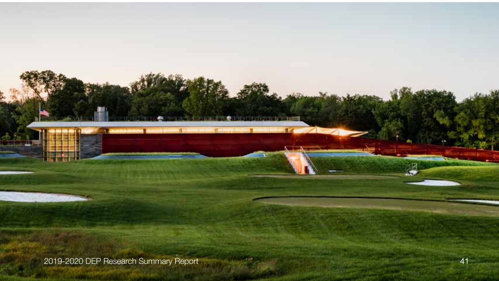
Croton Water Filtration Plant
