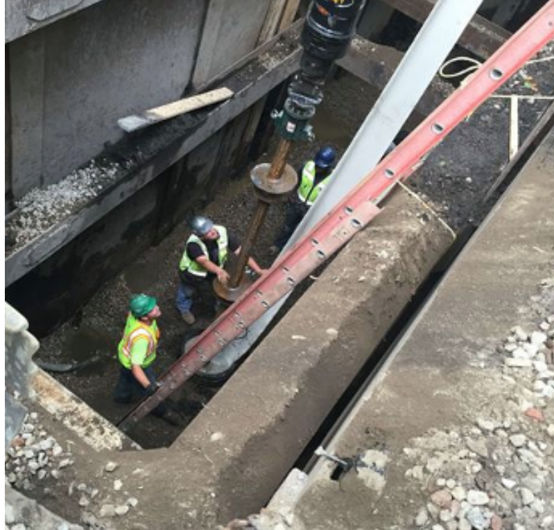
Installing DriveCast Helical Piles (DCP) at DEP work location.
