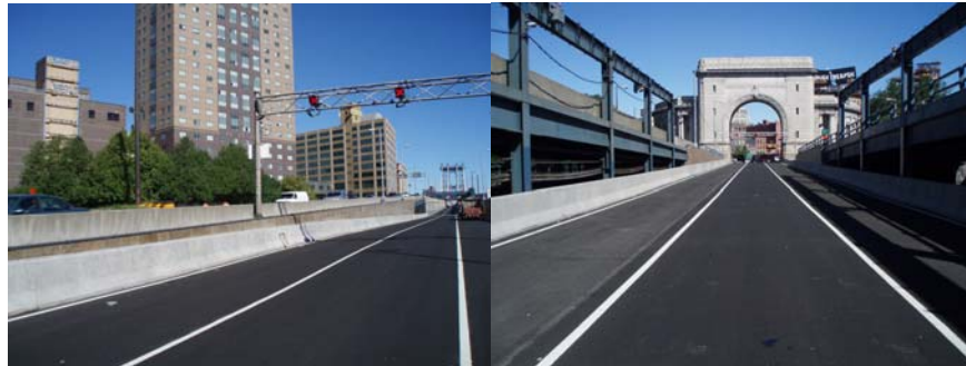
The Completed Lower Roadway on the Brooklyn Side And Near the Manhattan Colonnade.
