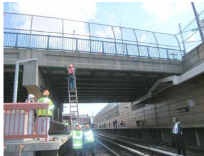
Inspecting the New Dorp Lane Bridge.
