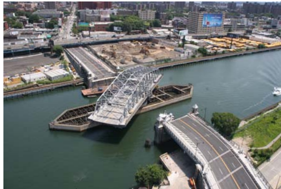
New 145 th Street Bridge Open for Marine Traffic.
