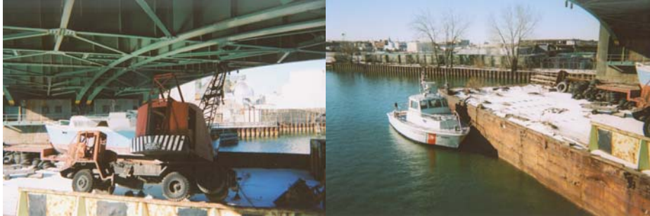
Barge Stuck Under the Greenpoint Avenue Bridge. Coast Guard Arriving to Investigate.
