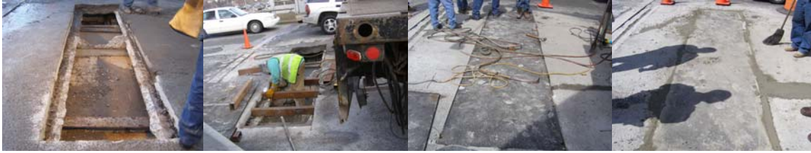
Willis Avenue Through-Hole Repairs. (Credit: Mohammad Awal)
