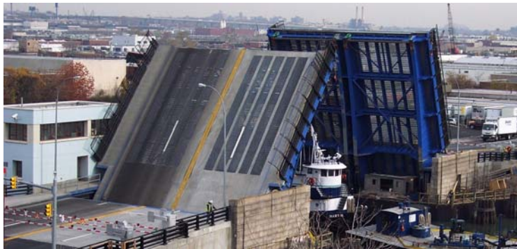
Tugboat Pushing a Barge Under the Open Metropolitan Avenue Bridge.
