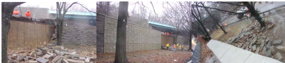
Inspecting the Mosholu Parkway Retaining Wall.
