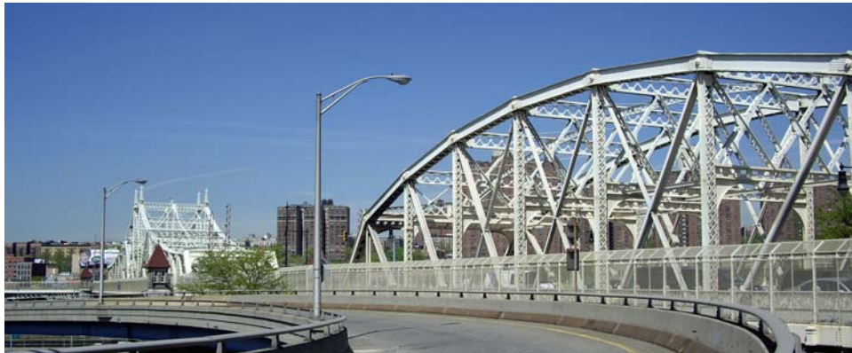
Macombs Dam Bridge in May 2007.
