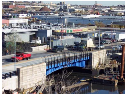
Northeast View of the Metropolitan Avenue Bridge.
