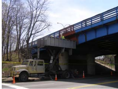
Painting Flatbush Avenue Bridge over Belt Parkway. (Credit: Earlene Powell)
