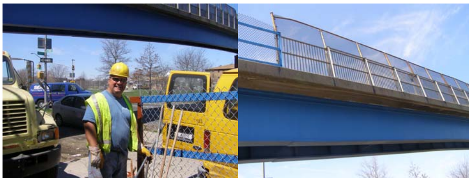
Bridge Painter Brian Kavanagh at the Whitelaw Pedestrian Bridge. Section of the Bridge. (Credit: Earlene Powell)
