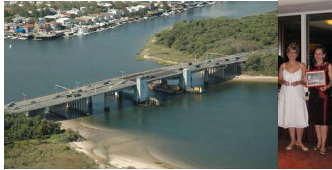
Aerial View of the Belt Parkway Over Mill Basin Bridge. Director of Design-Build/Emergency Contracts Chris Sklavounakis and Deputy Director of Design-Build Beatriz Duran at the Award Ceremony.
