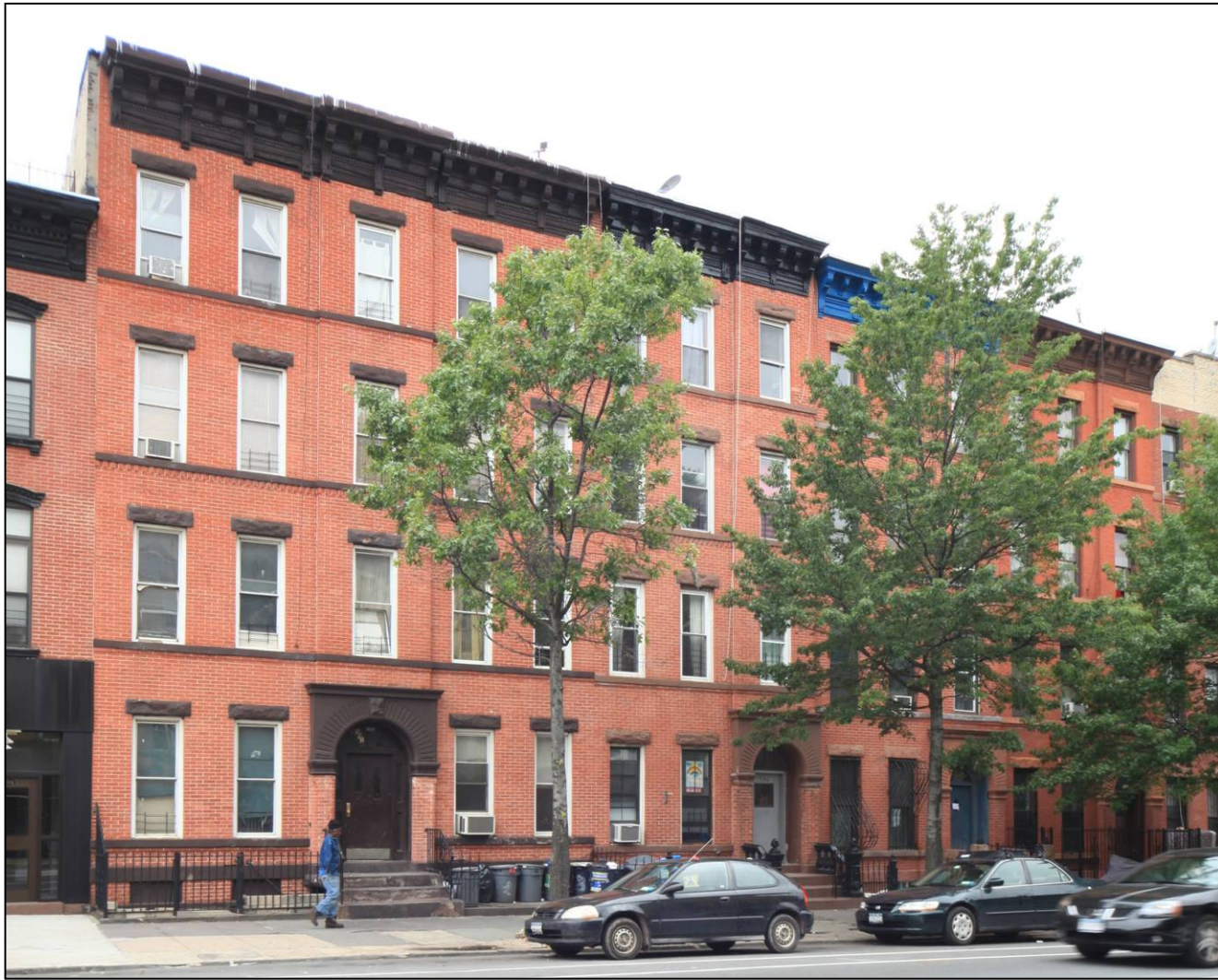
Figure 22 592-586 Vanderbilt Avenue Timothy Remsen, No. 578-588, c. 1891; No. 590-592, c. 1894 Photo: Christopher D. Brazee
