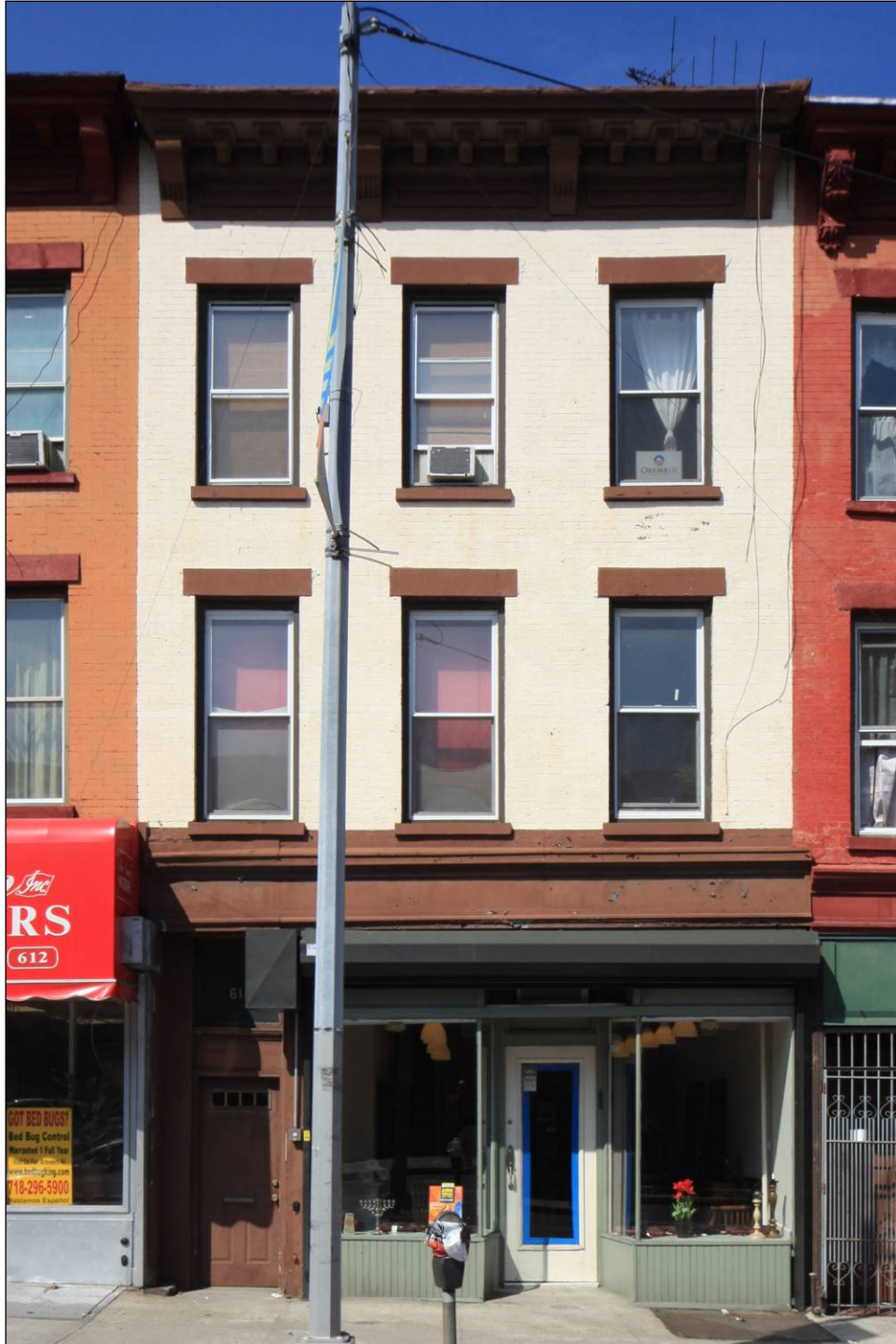
Figure 17 610 Vanderbilt Avenue Architect not determined, c. 1871 Photo: Christopher D. Brazee
