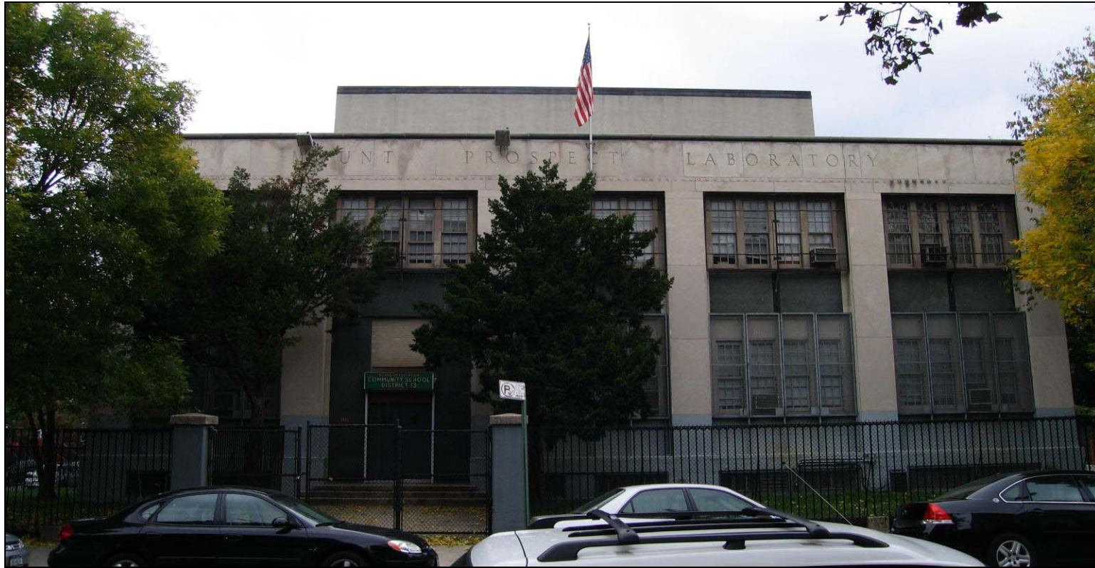
Figure 33 Former Mount Prospect Laboratory Building 349-355 Park Place aka 147-151 Underhill Avenue Aymar Embury II, c. 1938 Photo: Donald G. Presa
