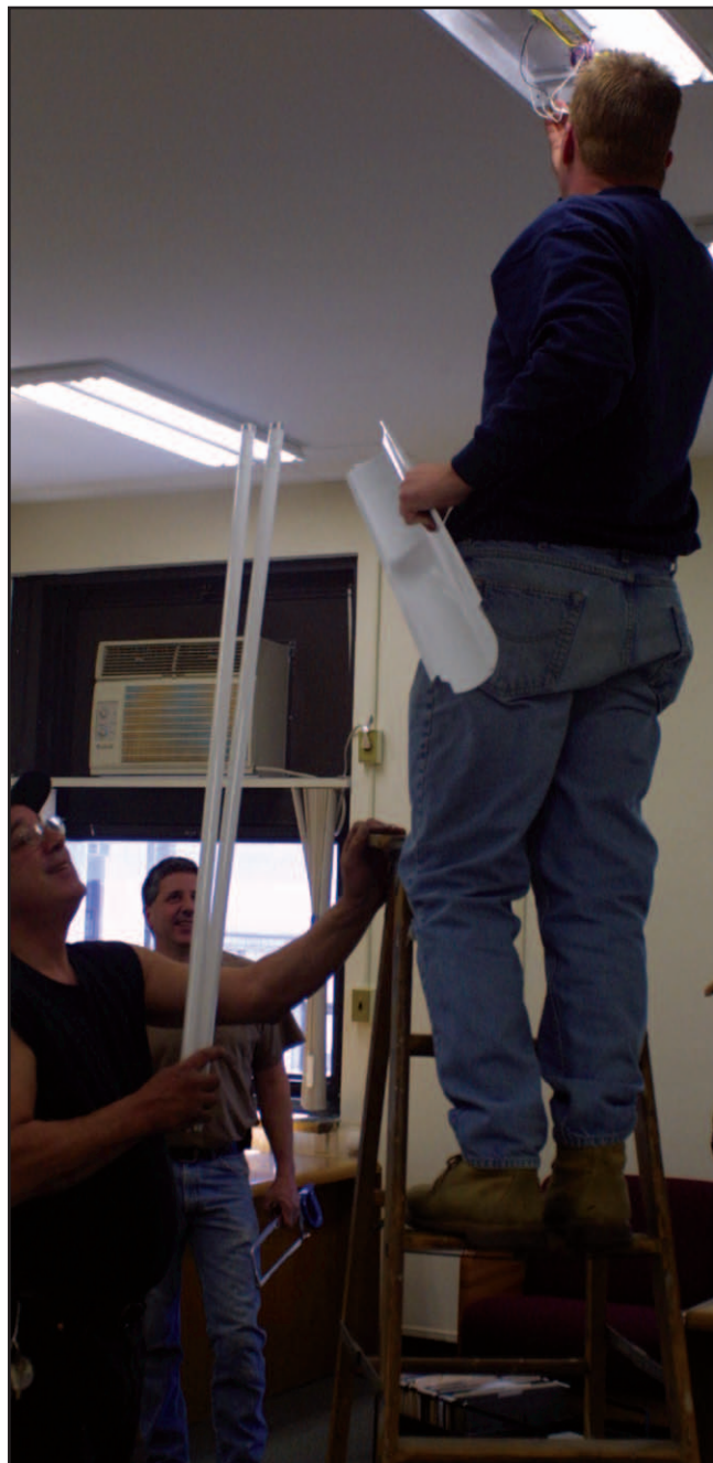
BBM Electricians repair light fixture
