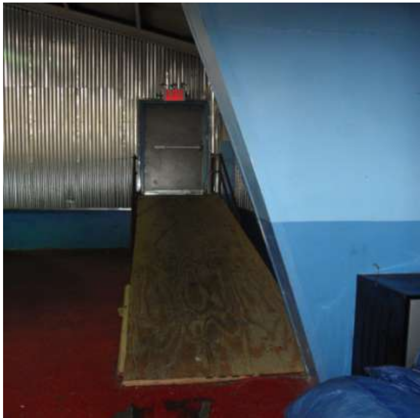
Ramp Covering Exit Stairs near Soccer Field
