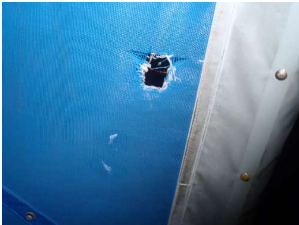
Damaged Indoor Jungle Gym
