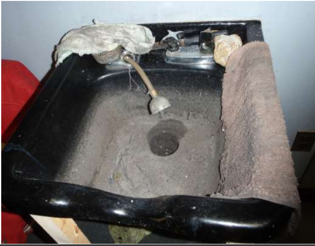
Unsanitary Sink in Massage Room
