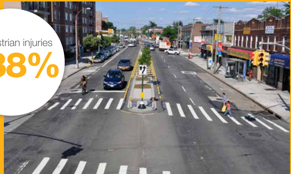
Hillside Ave at 187th St (after)
