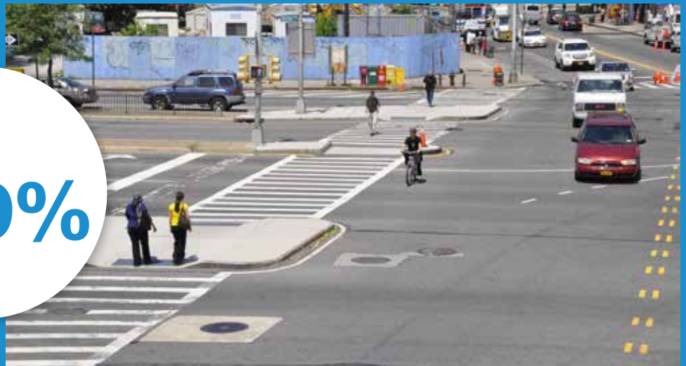
Queens Boulevard at Broadway (after)
