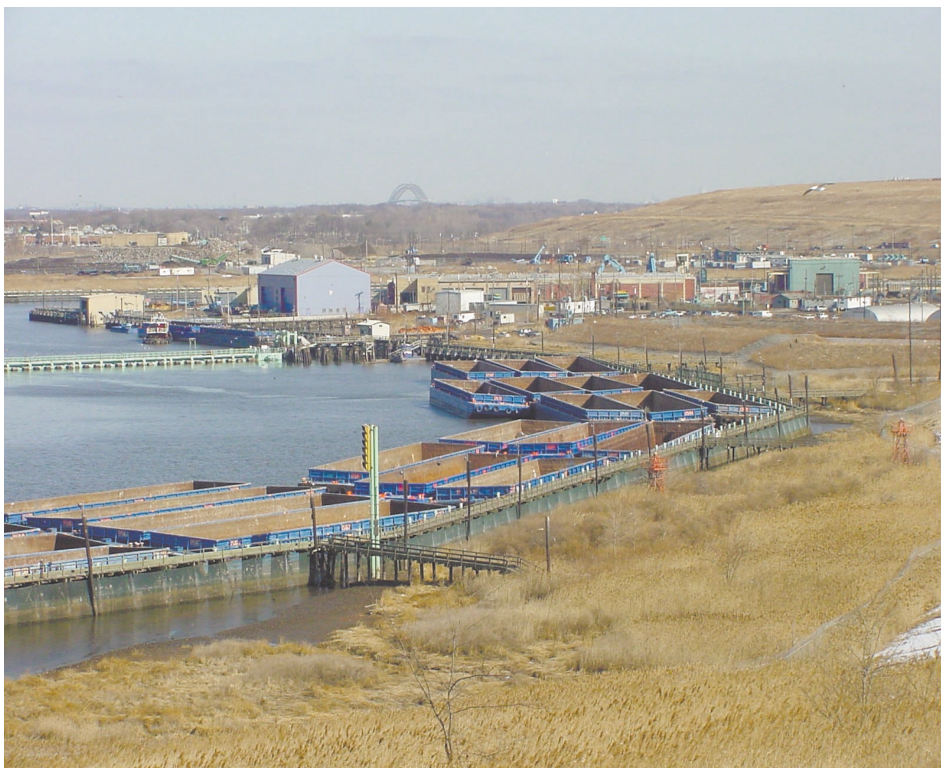
View of barge staging area from Sections 1/9 at Fresh Kills Landfill.
