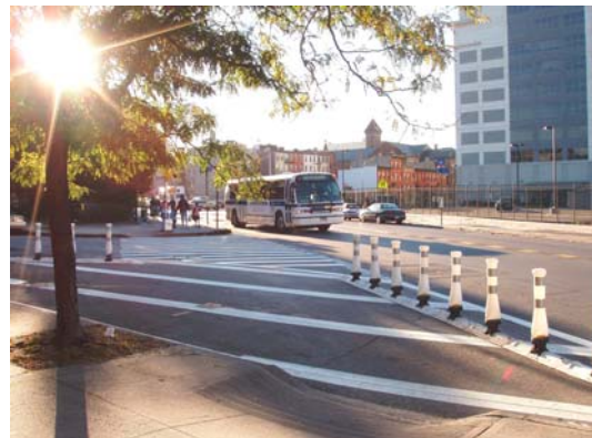
Figure 2. After. Looking east on Fulton Street at Gates Avenue.
