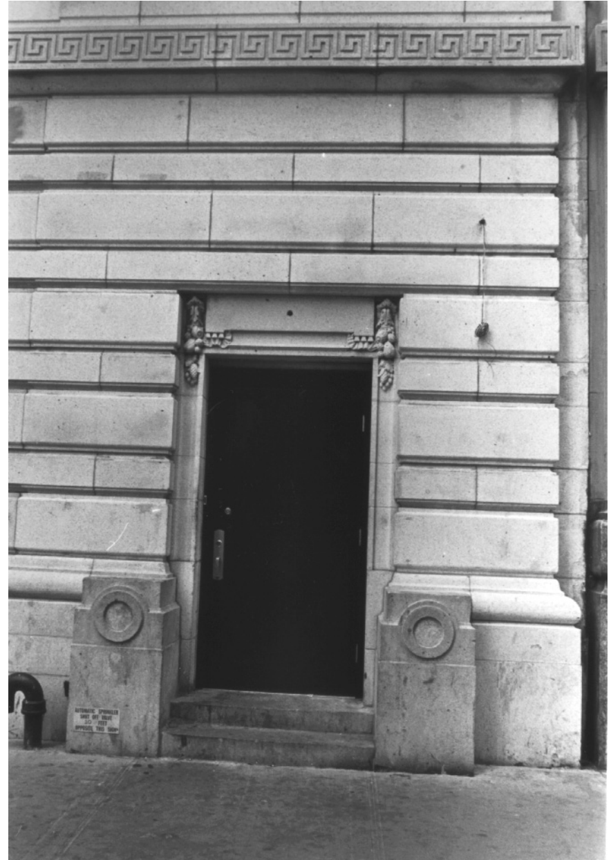
American Bank Note Company Office Building Rear door on Beaver Street Photos: Carl Forster
