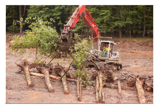
Constructing the base of the new stream bank with root wad revetment.
