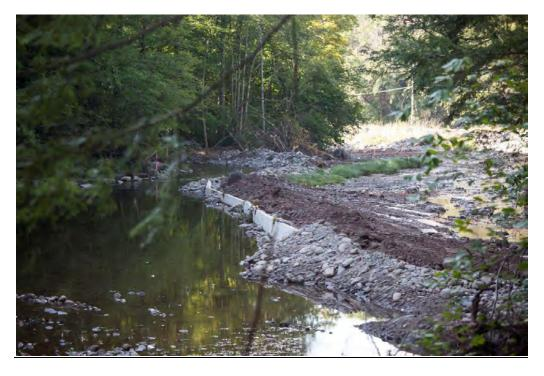
Coffer dam installation to create bypass channel; diverts stream around project site.
