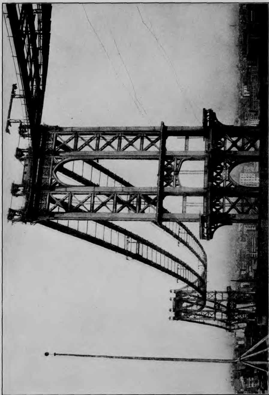
MANHATTAN BRIDGE—Towers and Completed Footbridges.
