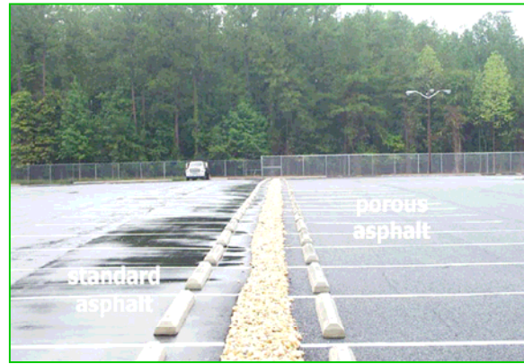
FIGURE 5.6 Porous bituminous asphalt - consists of standard bituminous asphalt in which the fines have been screened and reduced, allowing water to pass through very small voids. Porous asphalt is suitable for use in any climate where standard asphalt is appropriate and its compressive strength is similar to conventional asphalt pavements; Source: Draft Pennsylvania Stormwater Management Manual, 2005
