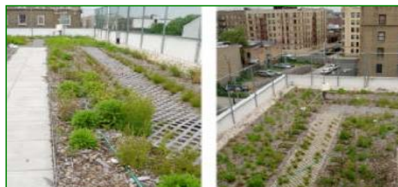
One of Gaia Institute's green roof projects in the New York City area; Source: Gaia Institute
