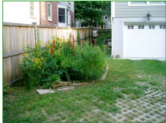
Attractive examples of residential BMPs including a rain garden on left and porous paver blocks on right. Source: Amy S. Greene Environmental Consultants
