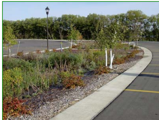
Vegetated swale installed in road median; Source: USDA Natural Resources Conservation Service
