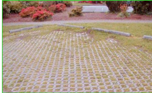
FIGURE 5.7 Porous paver blocks - Porous paver blocks consist of interlocking units (often concrete) that provide some portion of surface area that may be filled with a pervious material such as gravel. These units are often very attractive and are especially well suited to plazas, patios, small parking areas, etc. The compressive strength of pavers varies depending on the product, but tends to be high (up to 8,000 psi); Source: Draft Pennsylvania Stormwater Management Manual. 2005
