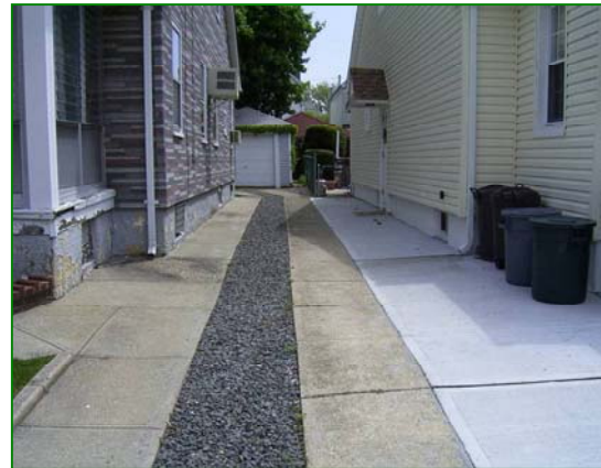
Permeable gravel parking strip in residential neighborhood of the Jamaica Bay Watershed; Source: Biohabitats
