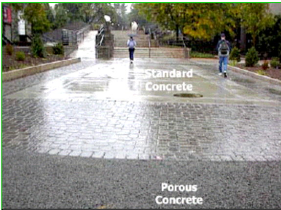
FIGURE 5.5 Porous concrete – Like porous asphalt, porous concrete is produced by substantially reducing the number of fines in the mix in order to establish voids for drainage. The pavement will support traffic and allow water to pass through to a gravel layer underneath. The strength of pervious concrete is about 85 percent of conventional concrete, making it suitable for sidewalks, driveways, alleys, parking lots and residential streets. In northern and mid-Atlantic climates, porous concrete should always be underlain by a stone subbase designed for stormwater management and should never be placed directly onto soil; Source: Draft Pennsylvania Stormwater Management Manual, 2005
