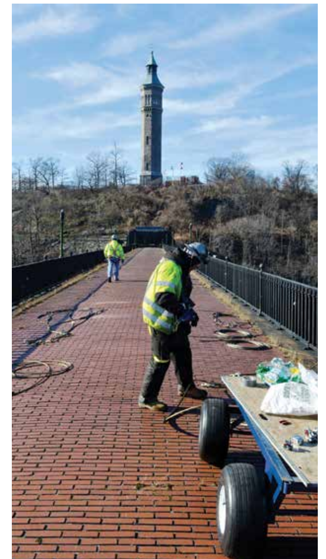
Top: Autumn in Fort Tryon Park, Manhattan. Bottom: Reconstructing the High Bridge between the Bronx and Manhattan.
