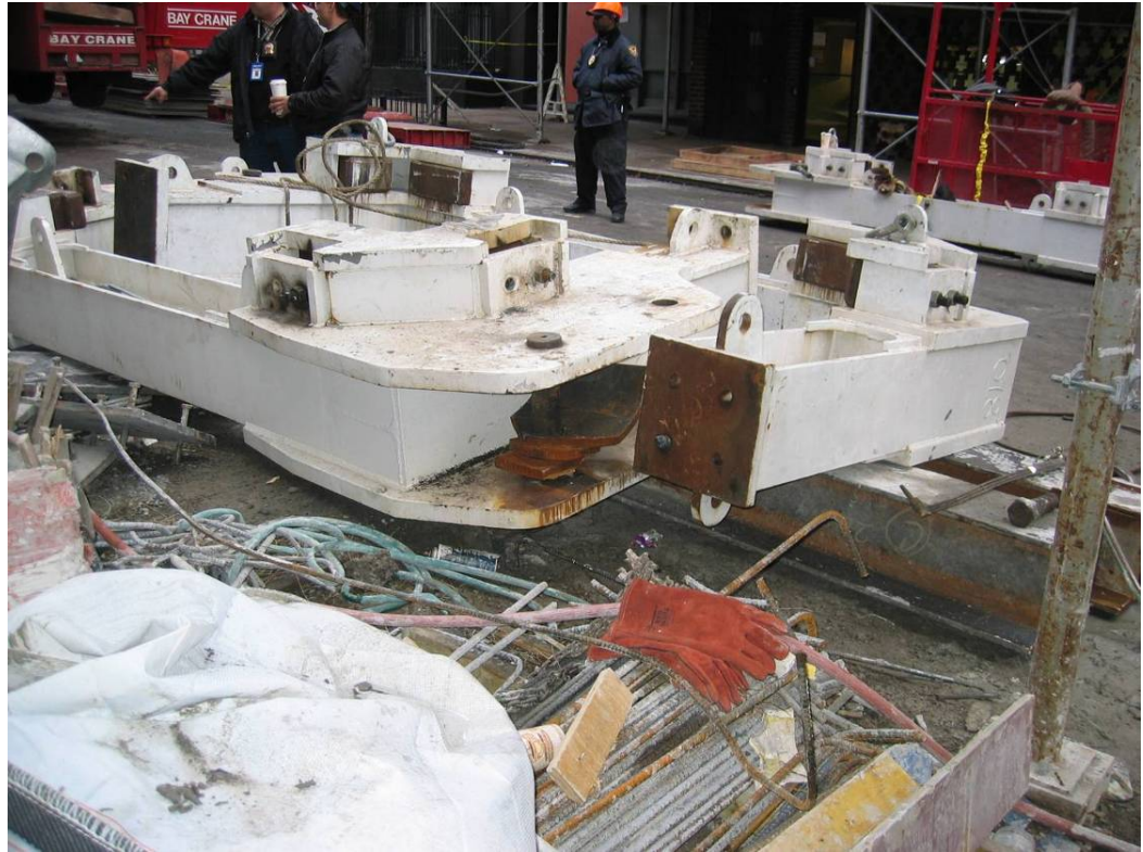
9 th Floor Collar Assembly
