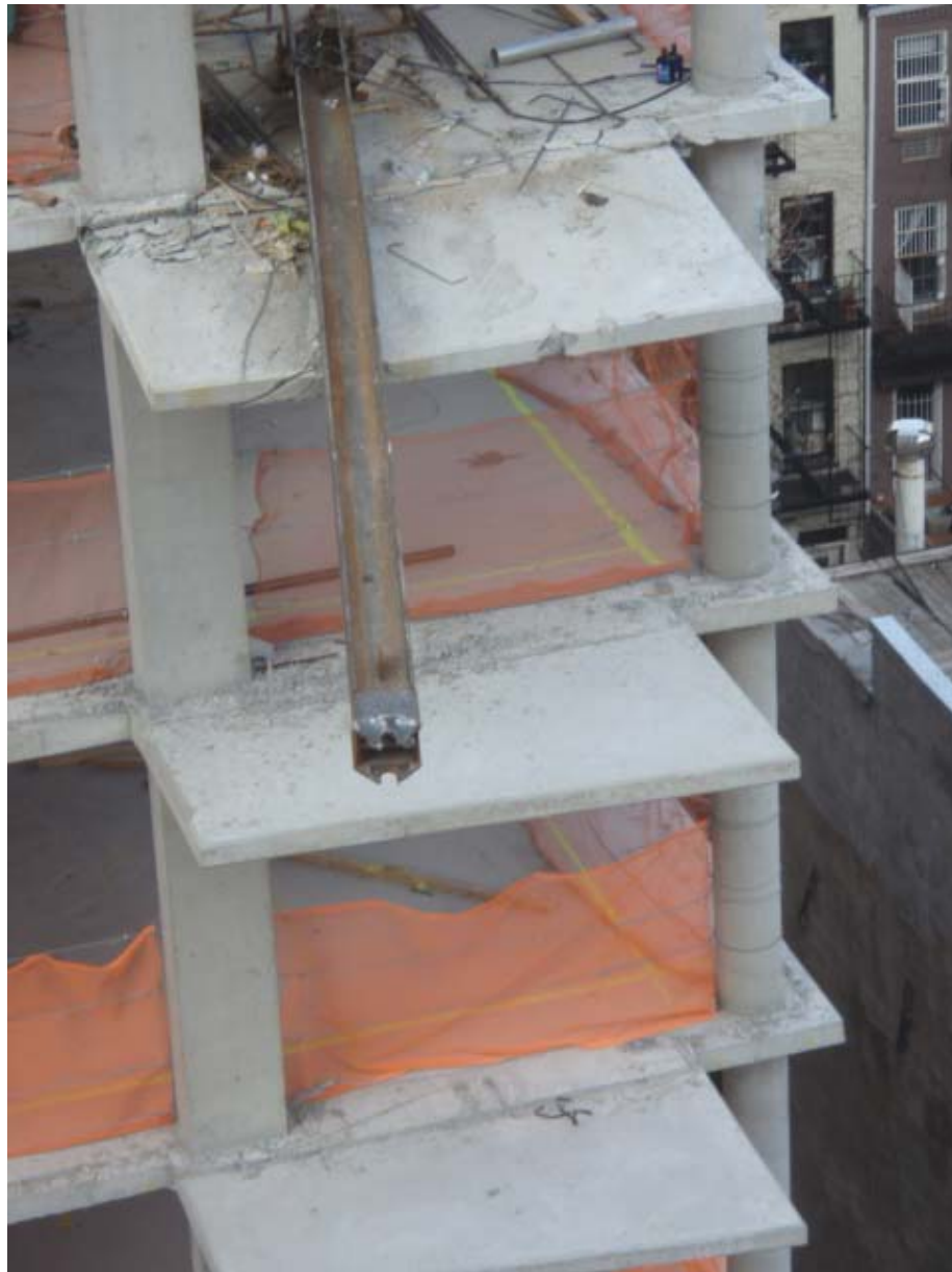
Photograph 1.13 - Failed pin end of Beam B5 at the 9 th floor level as seen immediately following the collapse. Photo provided by the NYCDOB.
