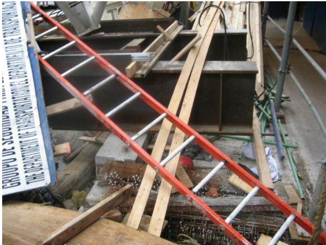
Photograph 1.17 - View of building side (north) of tower base after collapse. The dunnage beam has been displaced towards the building and the plywood bearing pads are off of the foundation wall. Lifting of the back tower legs and slippage of the front tower legs is also visible. Photo by New York County District Attorney IMG_379_109.jpg.
