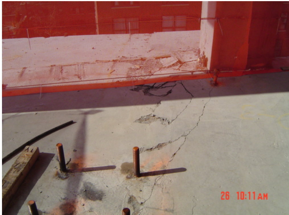
Photograph 1.20 - Minor spalling of concrete in the vicinity of the bolted connections to the 9th floor slab. Photo by Arup.
