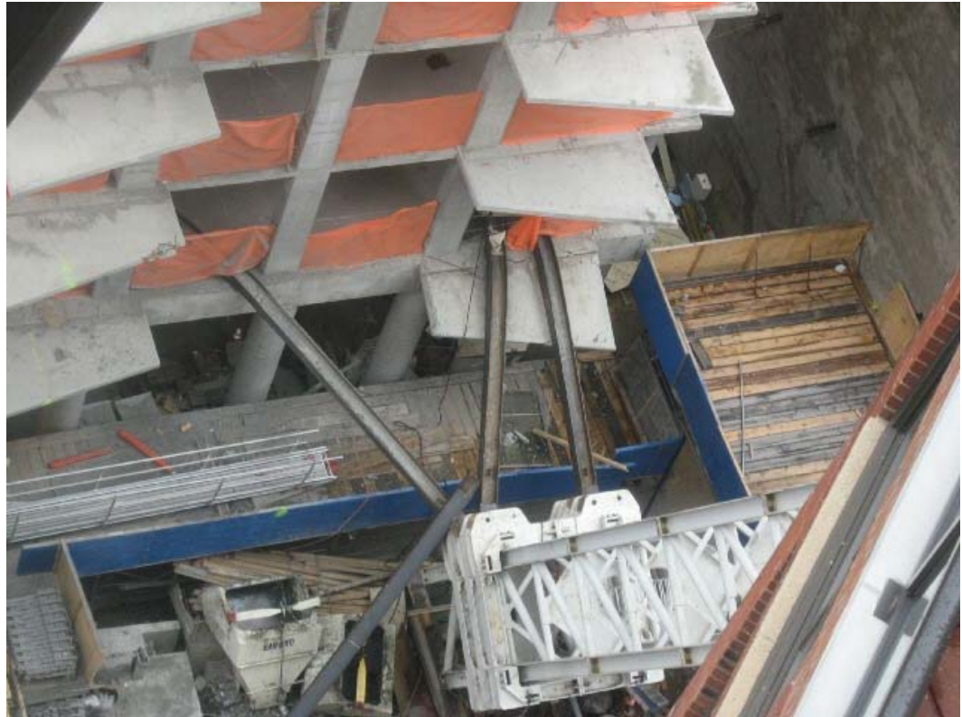
Photograph 1.14 - 3rd floor collar assembly following the collapse. The 9th floor collar and 18th floor collar rest atop the 3rd floor collar. Source: New York County District Attorney IMG_0355_085.jpg.
