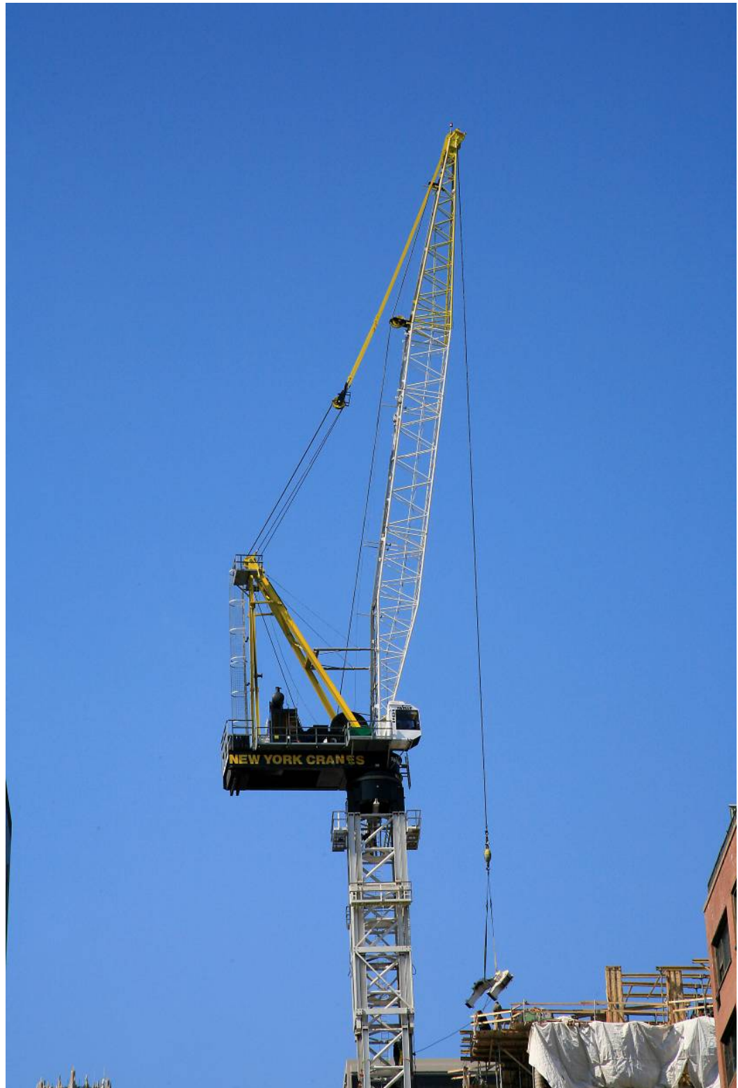
Photograph 1.7 - Photograph showing the position of the crane boom during tie-in assembly, approximately 1 hour before the crane collapse (source: photograph by Gary Halby).
