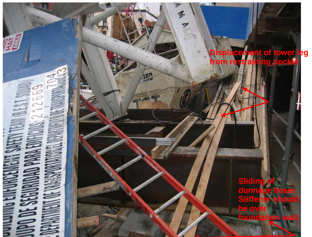
Photograph 11.3 - Base of tower crane after collapse. Note the movement of the dunnage beam and displacement of the tower legs from their restraining pockets. Photo from New York County District Attorney IMG_0379_109.jpg.
