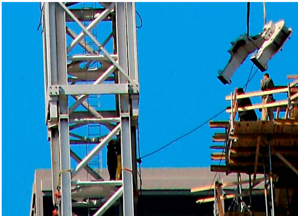
Photograph 8.1 - View of tower crane with collar half being lifted into place via polyester web slings attached to improper lifting lugs resulting in a non-horizontal position of the collar half during lift (right of photo) and chain falls incorporating polyester web slings choke hitched around the tower legs. (Source: photograph by Gary Halby).
