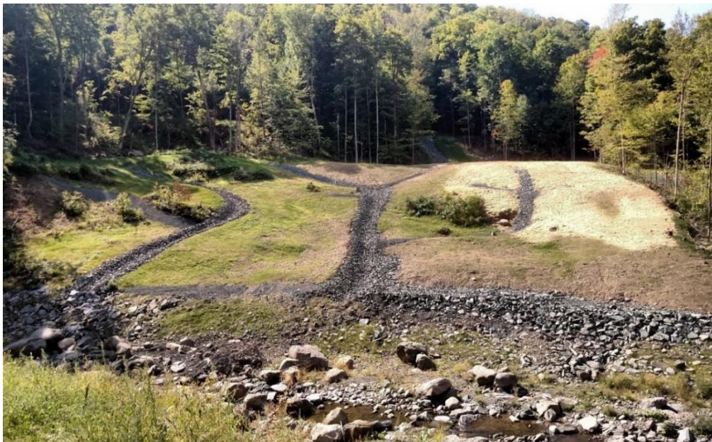
Figure 4.18 Wright Road site after construction.
