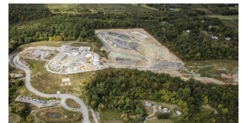
Figure 9.2 Aerial view of the Shaft 5B site.
