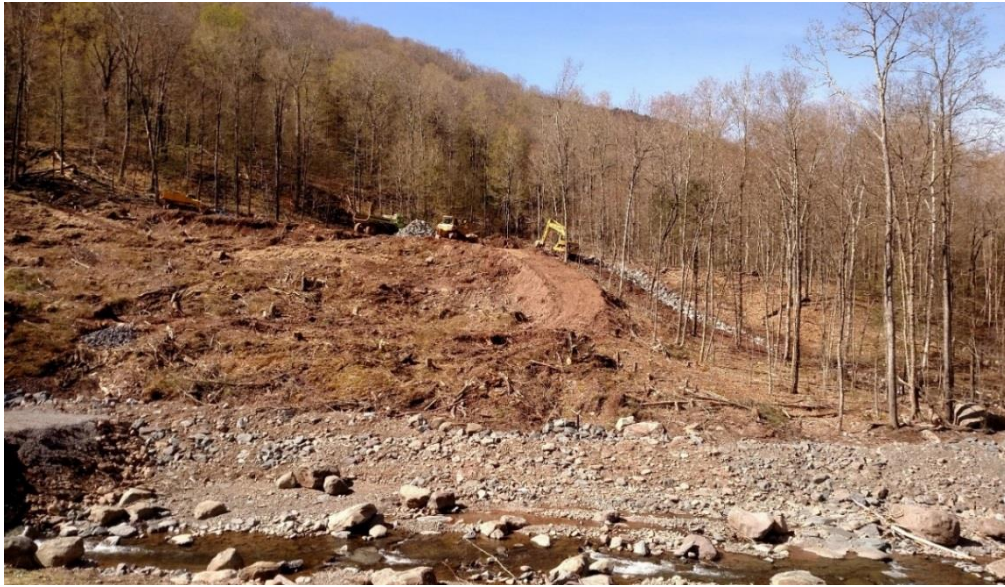
Figure 4.17 Wright Road hillslope before construction.
