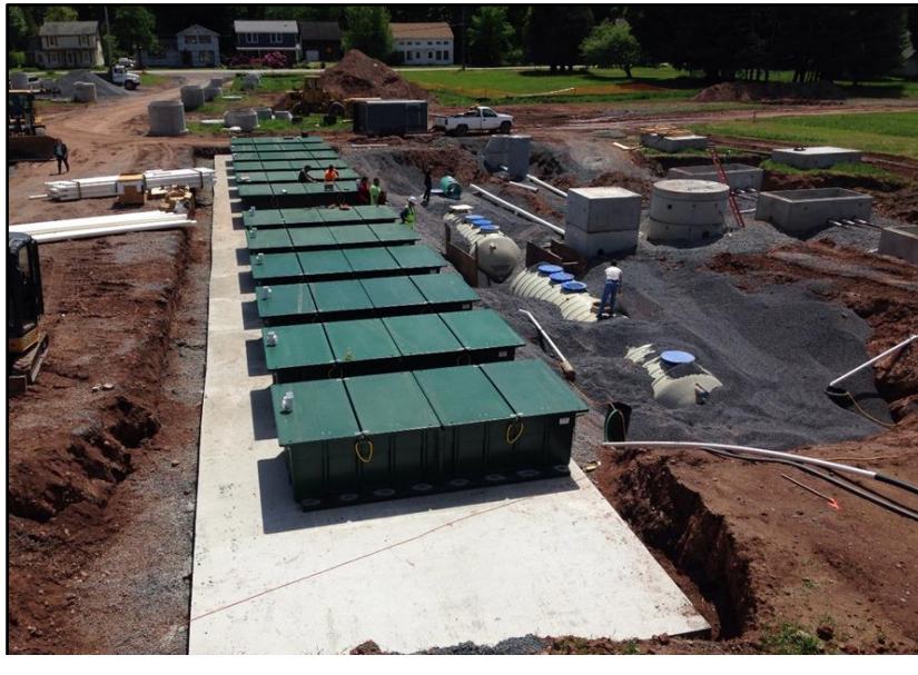
Figure 3.1 Installation of Orenco treatment units in Lexington.
