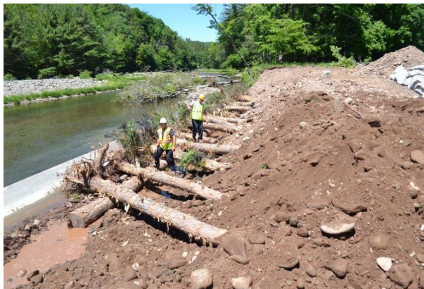
Figure 4.23 Installing root wad revetment.
