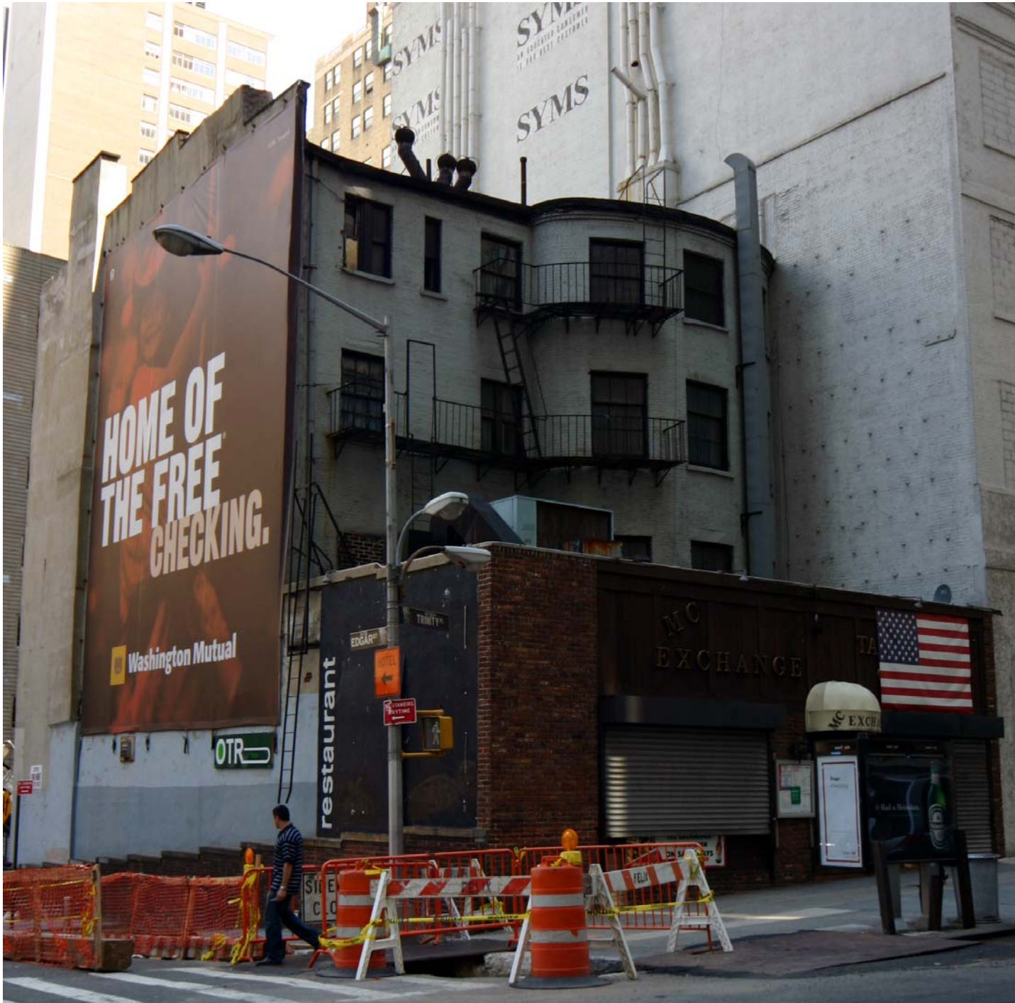
Robert and Anne Dickey House, rear and south façades Photo: Jenny Staley, LPC
