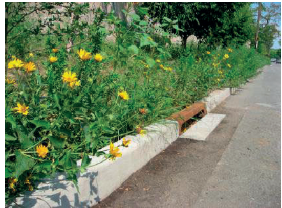
Low Density Residential Street: Post-Construction Infiltration Swale
