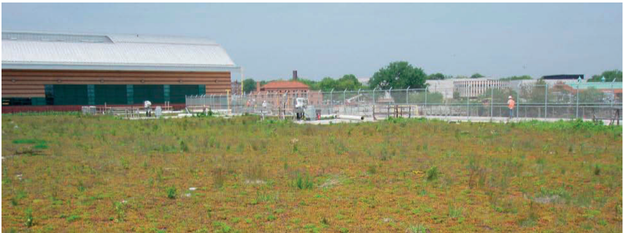
Figure 16: Green Roof at DEP's Paerdegat Basin CSO Detention Facility
