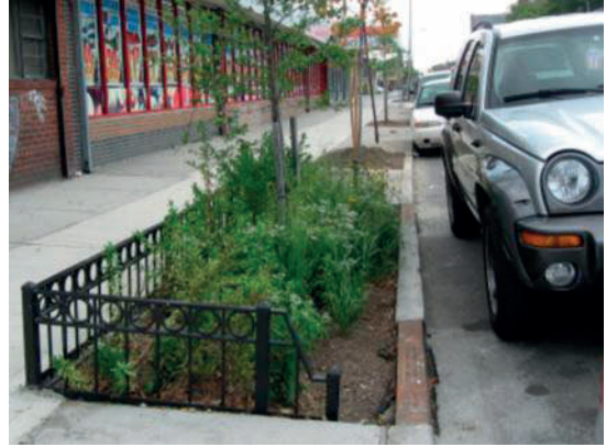
Commercial Corridor: Post-Construction Enhanced Tree Pit
