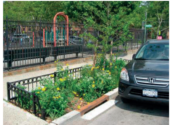
Low Density Residential Street: Post-Construction Enhanced Tree Pit
