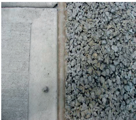
Figures 23: Pilot - Porous Concrete Sidewalk at DEP's Paerdegat Basin CSO Detention Facility
