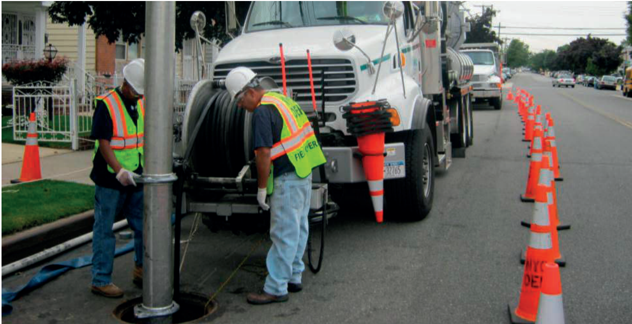
Figure 13: DEP Crew and Vactor Truck in Operation
