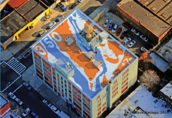
Artist Molly Dilworth created a cool roof for a school in Brooklyn. Dilworth painted a light-colored representation of the New York and New Jersey coastline after a 7 meter rise in sea levels.
