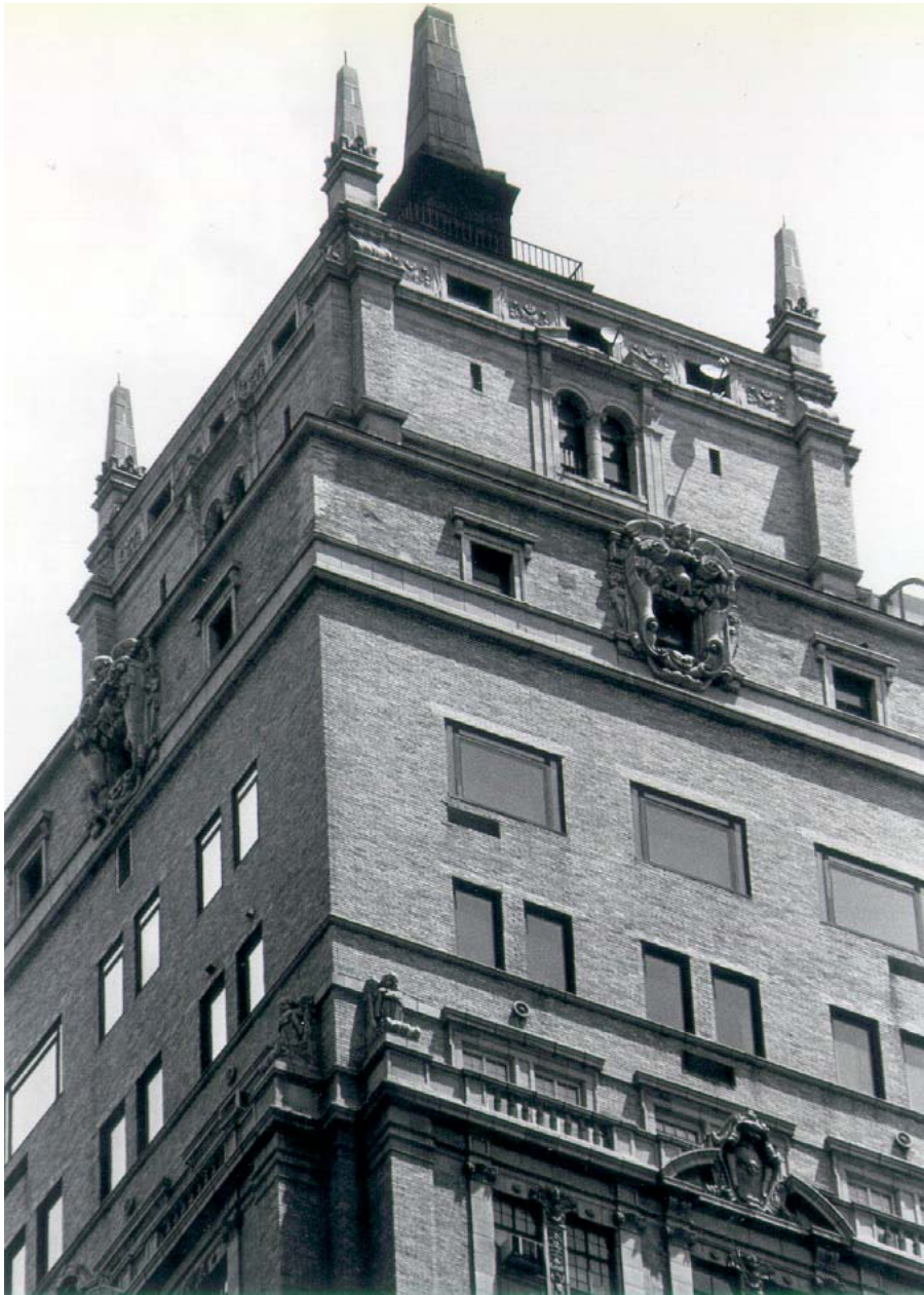
Roof detail, southern facade
