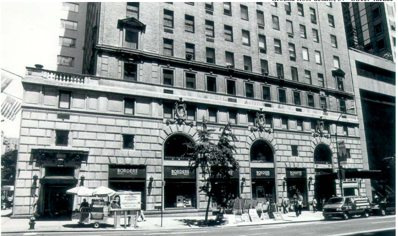
Ground floor details, 57 th Street facade
